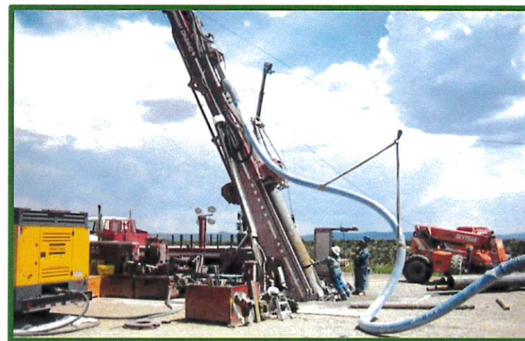
Drilling angled injection well for Interim Measure
