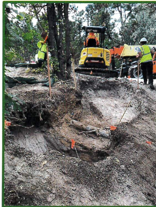
Sampling and cleanup of contaminated soil at a former outfall in TA-50, SWMU 50-006(d), and site stabilization after cleanup.
