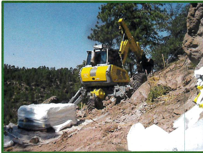
Excavation using a spider excavator at SWMU 01-001(d3)
