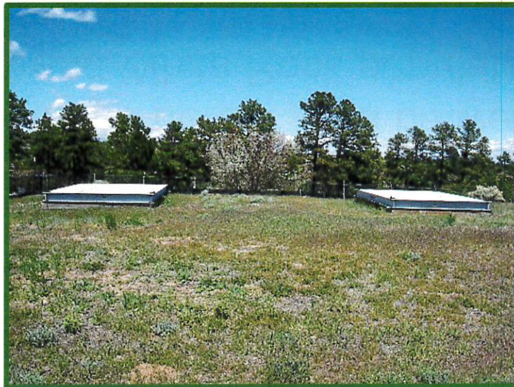
Material Disposal Area A
