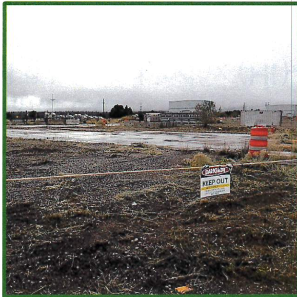
Remaining slabs at DP West at Technical Area 21 will be removed and sumps and waste lines investigated.
