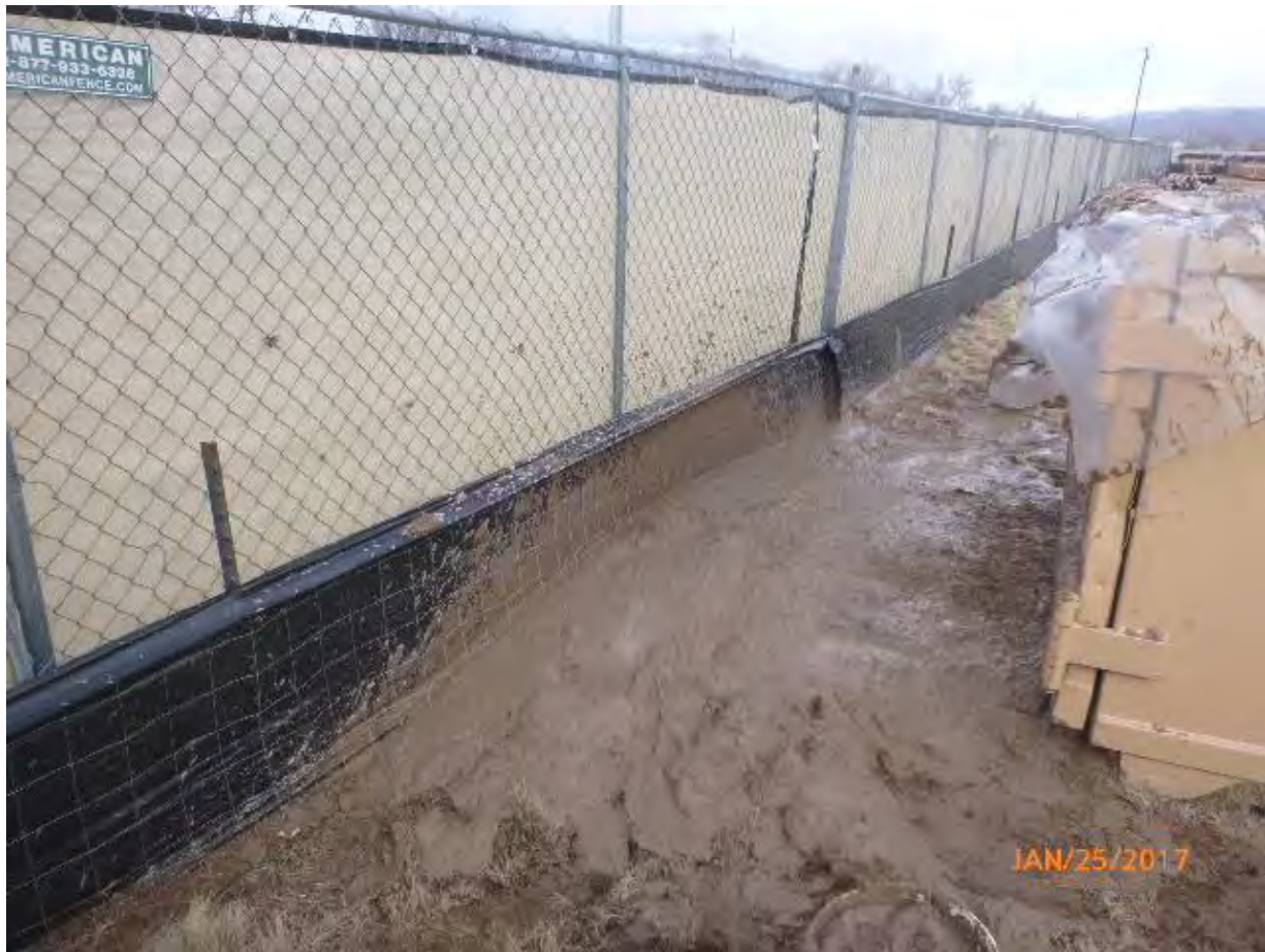
Photo 1. Site immediately after semi-saturated soil spilled, looking east.
