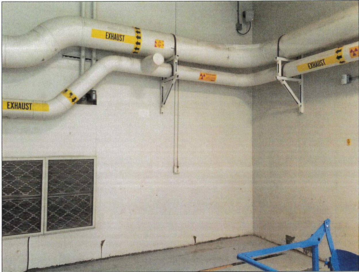
Photograph 1 Northeast Corner, Building 6580, Room 112 Sandia National Laboratories/New Mexico
