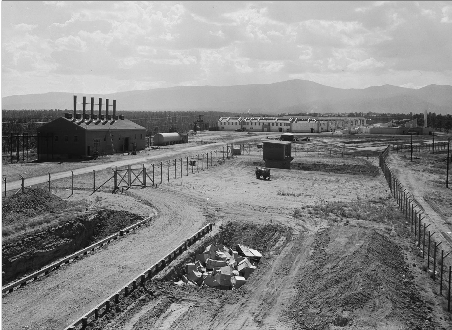
Figure 2.4-2 Waste disposal practices at MDA A circa late 1945; similar trench conditions and waste disposals are assumed to have existed at MDA B during this time period (LANL photograph IM-9: 2284).
