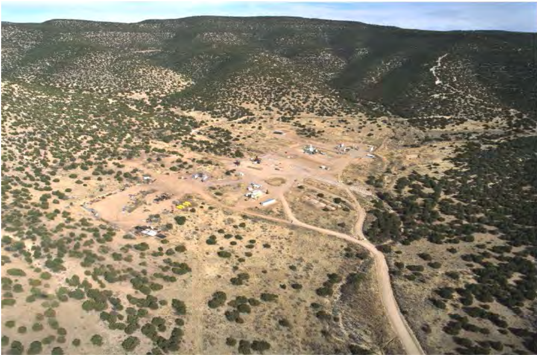
Burn Site Air Photo Looking North East
