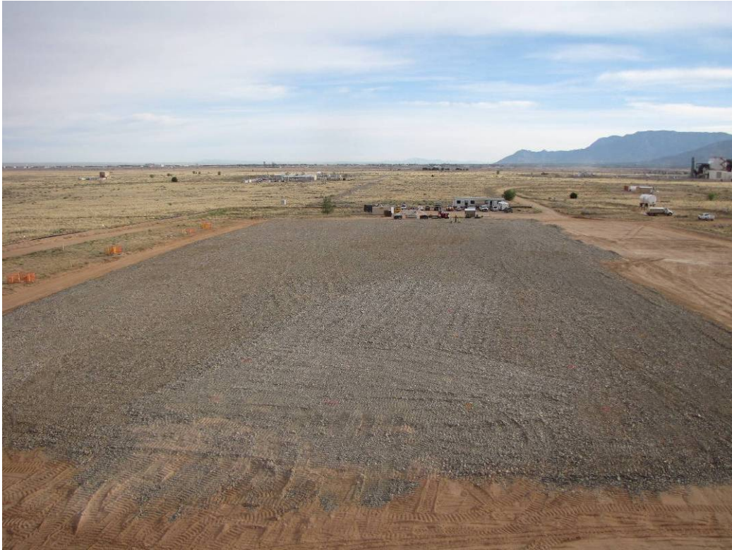
Bio-intrusion Rock Layer on June 8, 2009. View to north from the south end of the MWL.
