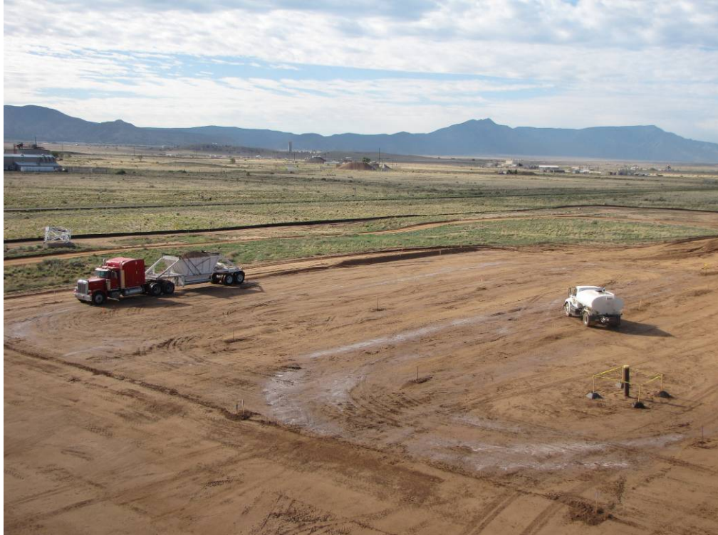
Bottom dump haul truck placing soil for Lift # 5 at northeast side of the MWL. View to southeast on June 30, 2009.
