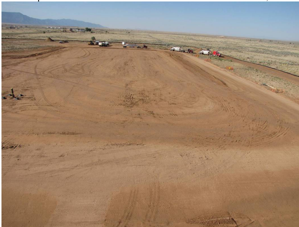
North slope completed to 6 to 1 slope and first 2 wedge lifts completed on east side. Lift #3 of Native Soil Layer in progress. View to the south on June 22, 2009.
