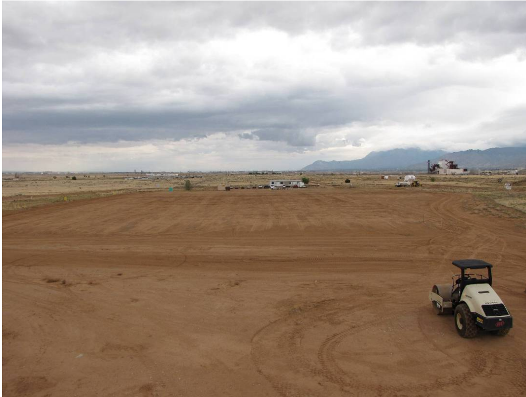
Subgrade Layer surface cleared, watered and rolled/compacted. View to the north from the south end of the MWL - May 26, 2009.
