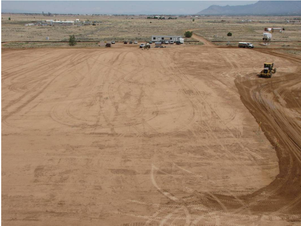
Soil Meniscus Layer (~3 inches thick) covering Bio-intrusion Rock Layer and slope work on east side of the MWL. View to north on June 18, 2009.
