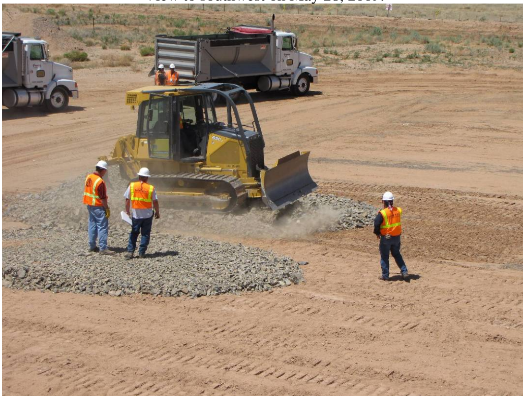
Spreading rock with bulldozer for Bio-intrusion Layer test. View to southwest on May 28, 2009.
