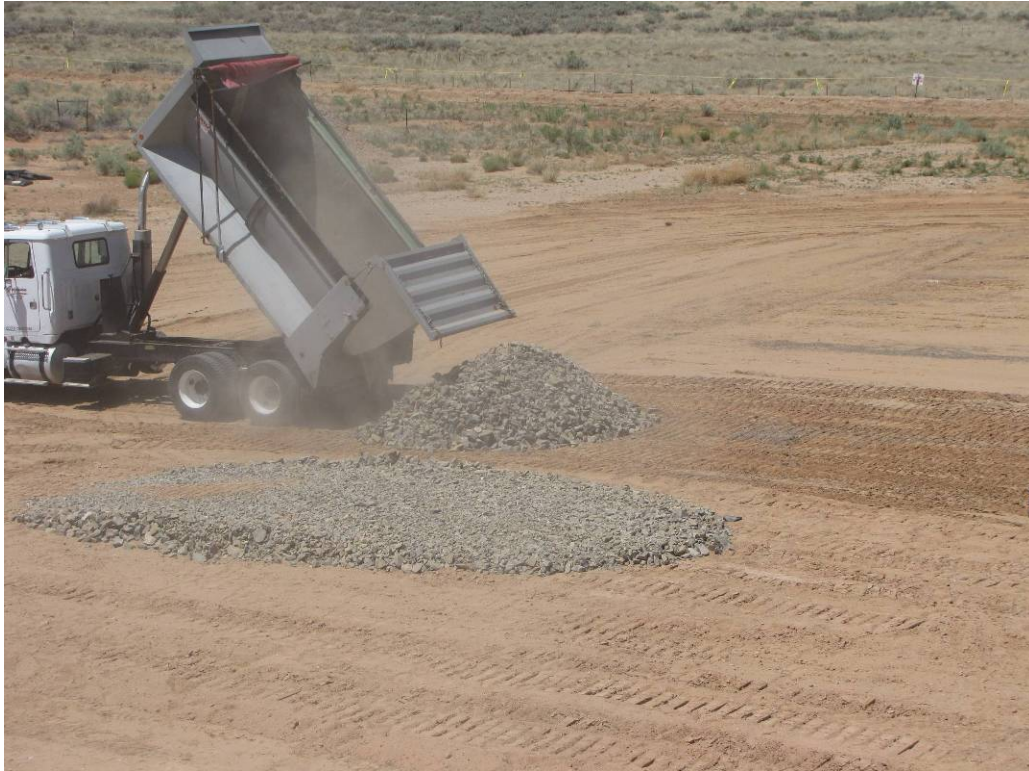
Start of Bio-intrusion Layer test at the south end of landfill. View to southwest on May 28, 2009.
