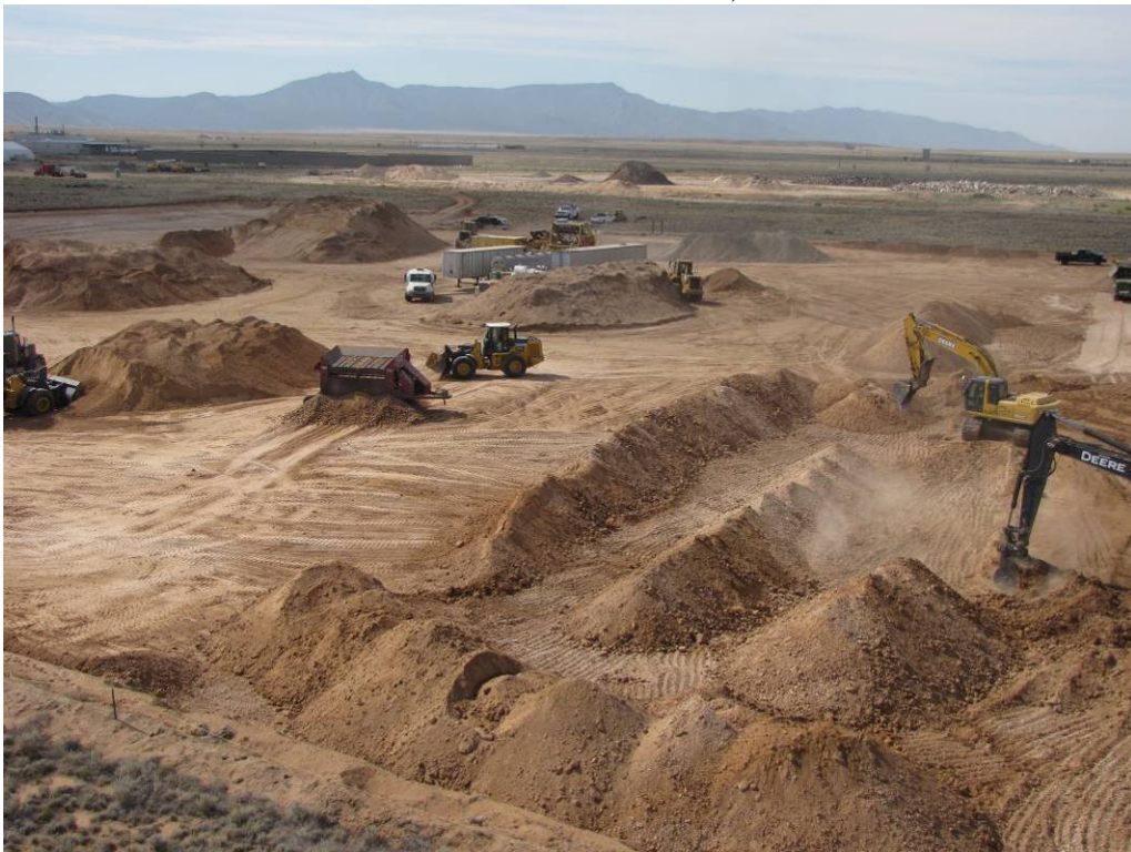
Borrow Pit Area activities on July 15, 2009. Pug Mill (background) and soil excavation and screening (foreground) operations. View to the south.
