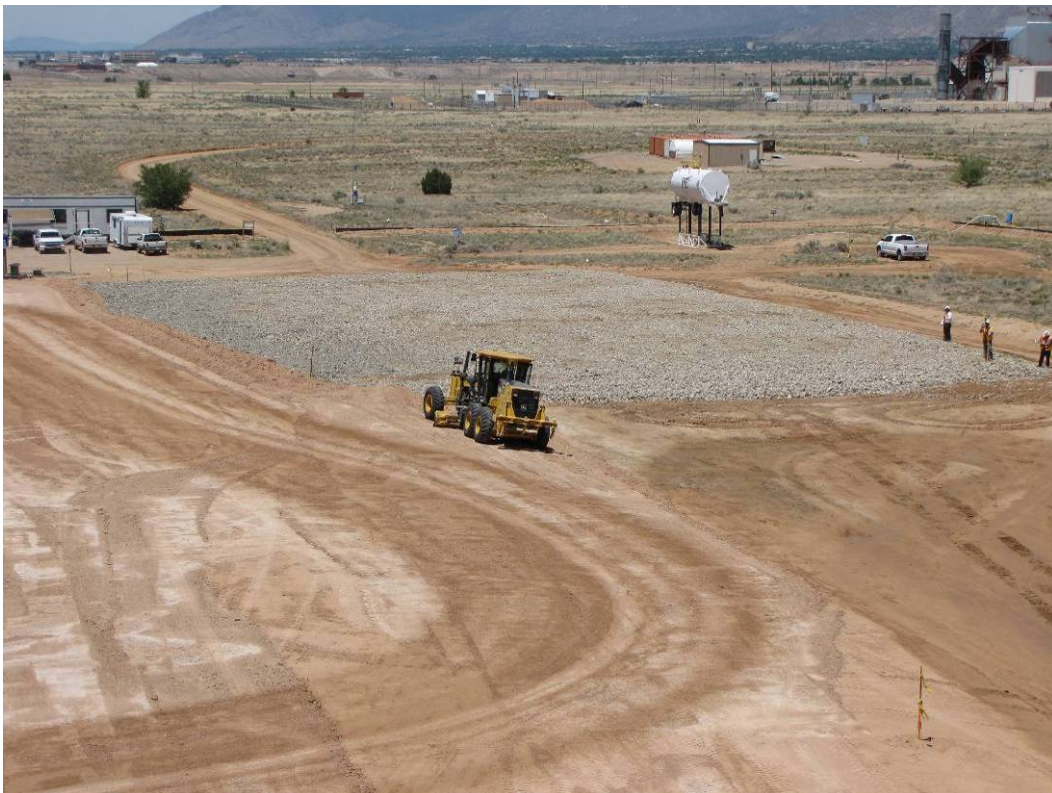
Completion of the Bio-intrusion Layer over the Classified Area – northeast end of MWL. View to north on June 12, 2009.
