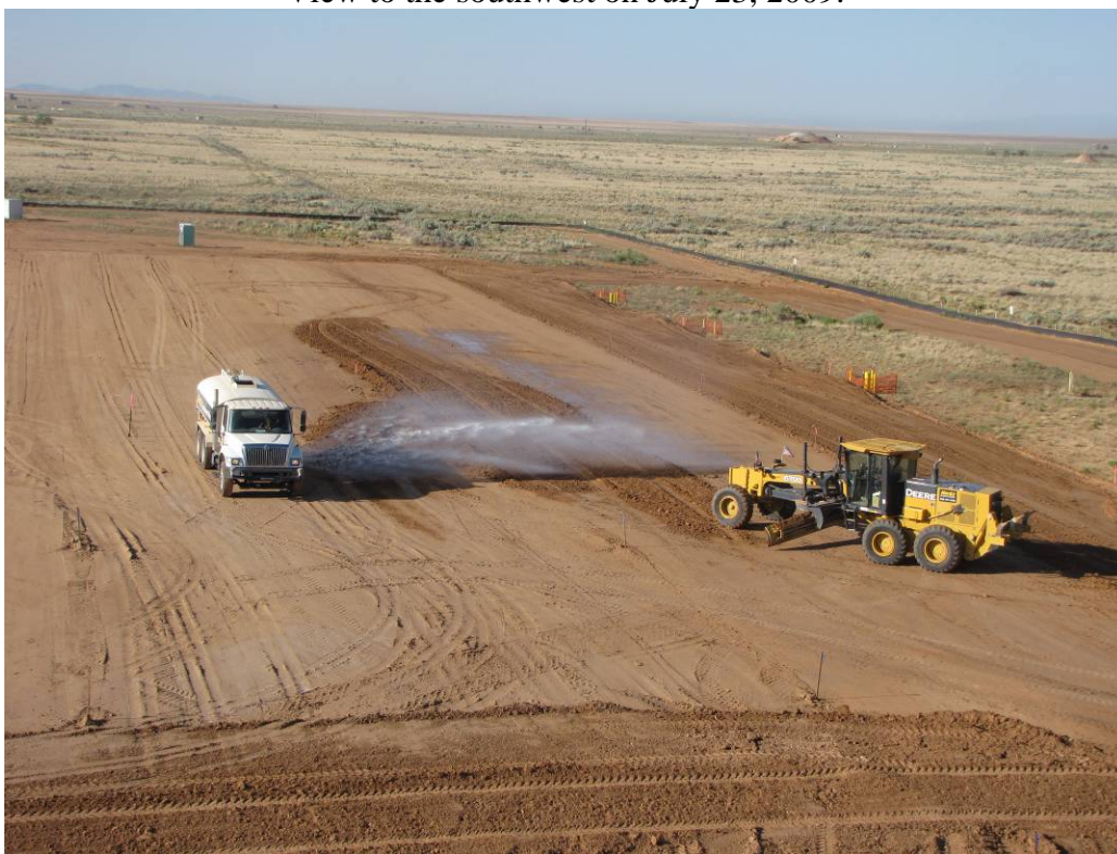
Soil being placed to adjust the Native Soil Layer thickness at specific grid points on the west side of the MWL after verification surveys. View to the south on July 31, 2009.
