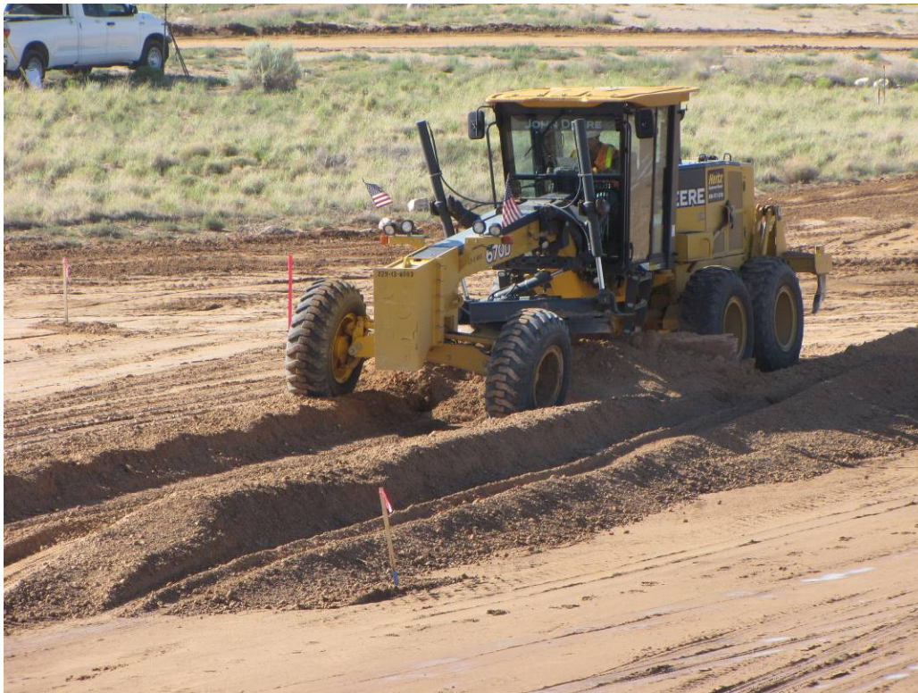
Motor grader spreading soil in dog leg area of MWL for Lift # 8. View to the southwest on July 23, 2009.
