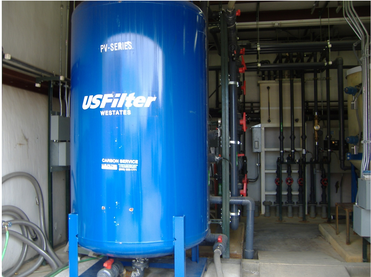
Photo E-11 Groundwater Treatment System, Carbon Unit
