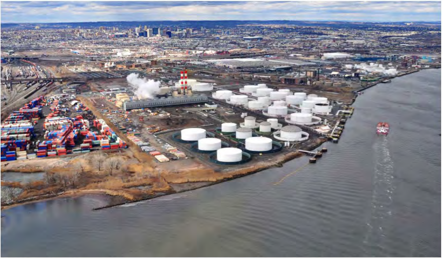
An aerial view of a biodiesel refinery and shipping facilities on the Passaic River waterfront with Newark, New Jersey, in the background.
