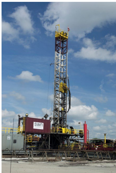
Figure 1-1 Typical rotary drilling operation- Source, Southwestern Energy
