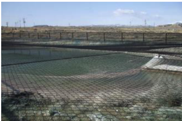
Figure 2-23: Netting over Impoundment
