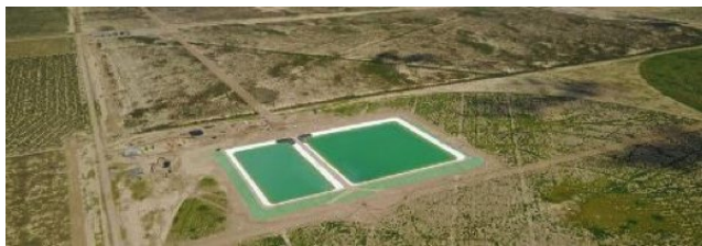
Figure 2-12: Layne Christensen’s Water Storage Facility in Reeves County, Texas
