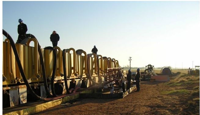
Figure 2-17: Frac Tanks Lined up Side by Side in Oklahoma
