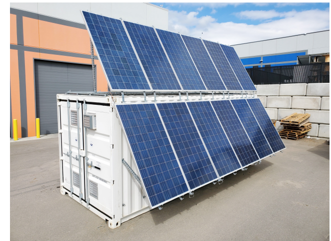
Hybrid solar & gas generation system designed to provide air and power for sites
