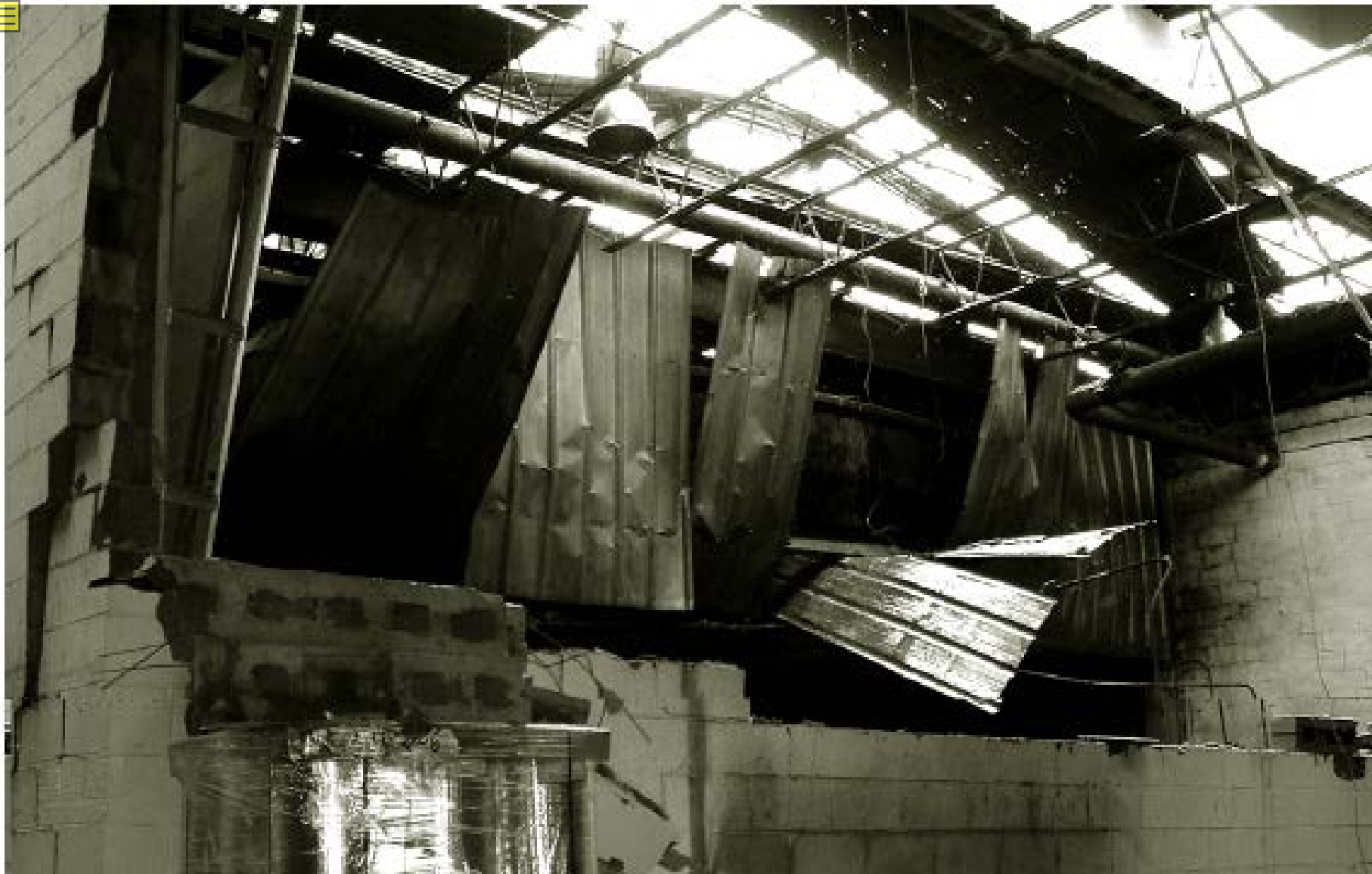
Collapsed firewall and metal panels – south end of line 405 blend room
