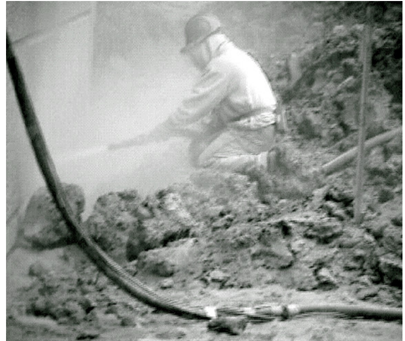
Figure 8. Worker performing abrasive blasting in an area with poor natural ventilation. The area was somewhat below ground level in sloping terrain. The dust exposure is obscuring the view of the abrasive blasting.
