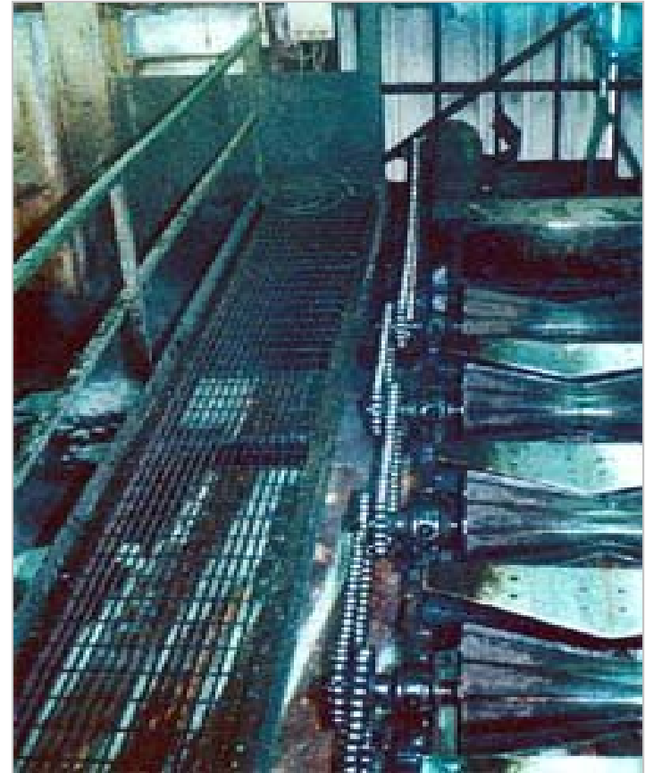
Roller conveyor with unguarded chain and sprocket drives
