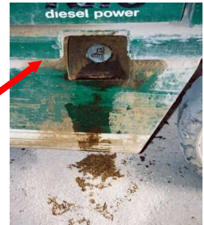
Fuel cap (note spilled gas on the outside of the truck.)
