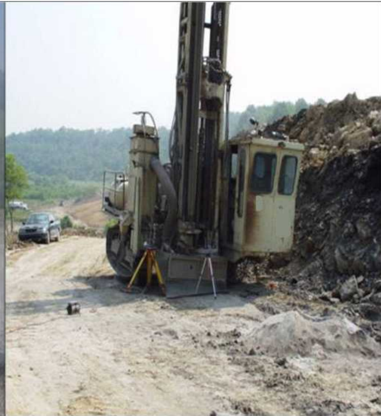
Wet drilling technique
