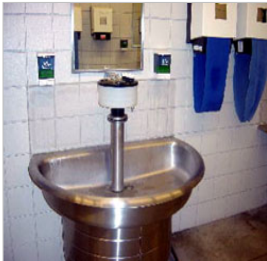
Hand wash station
