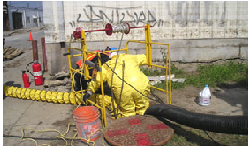
Photo courtesy of OSHA. This picture shows actual disaster site work conditions and may not illustrate proper safety and health procedures.
