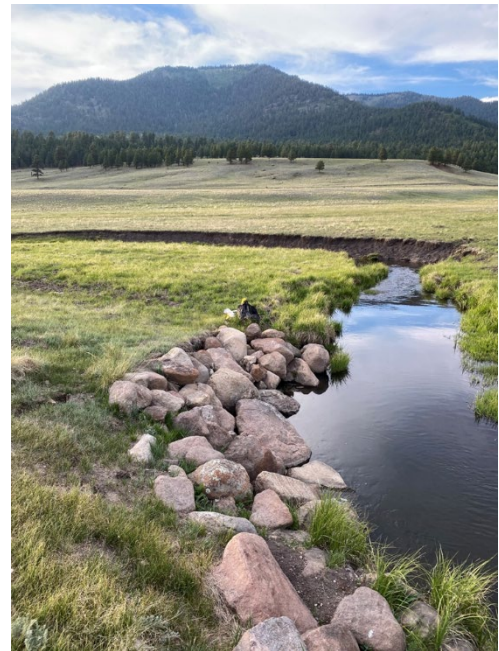
Rock armor to protect the road crossing at San Antonio creek above VC02 (stream temperature monitoring location)
