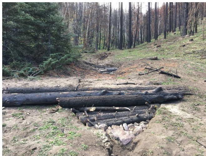
b) Post Fire Rehabilitation of the Rio en Medio: The completed structure.
