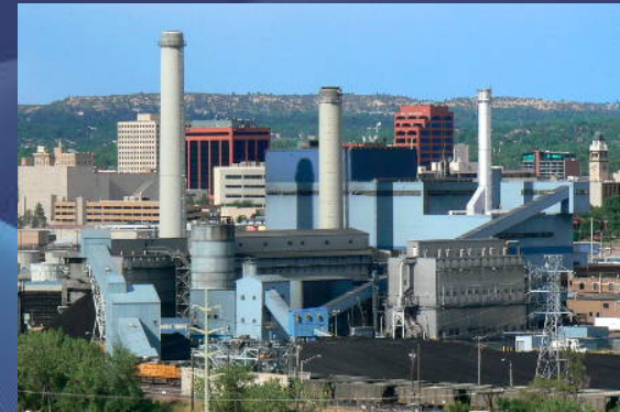
Martin Drake Power Plant
