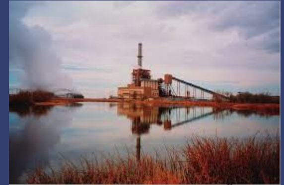
Pawnee Power Plant
