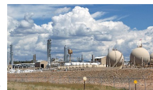
Natural Gas Processing Plant
