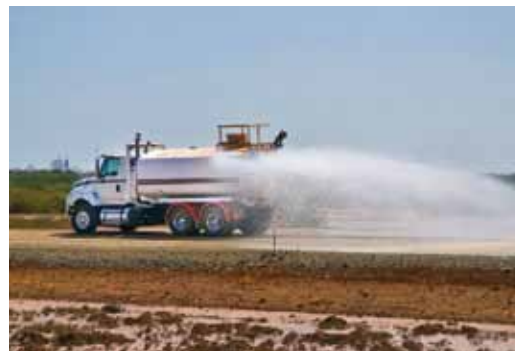
Figure 12: A water truck applies a chemical binder to the road.
