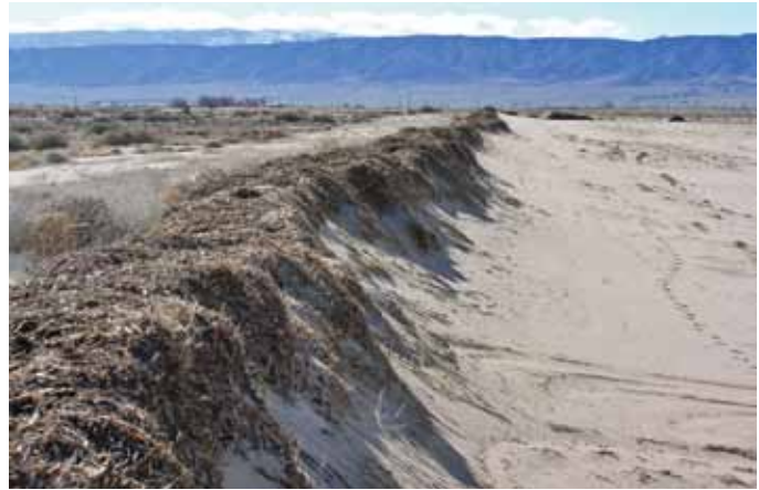
Figure 7: Berms are semi-permanent features on the landscape that provide effective reduction of blowing sand. (Prevailing wind blows from right to left.)
