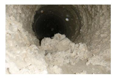
If air velocity in baghouse intakes falls below the minimum require to keep dust in suspension it will settle out and restrict air flow even more.
