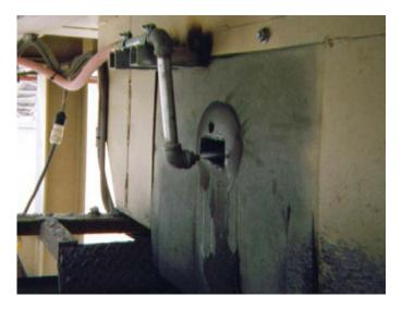
Protect nozzles from deposition that can plug them up by installing a dust curtain that protects them from the "blowback" of mist and wet fines.
