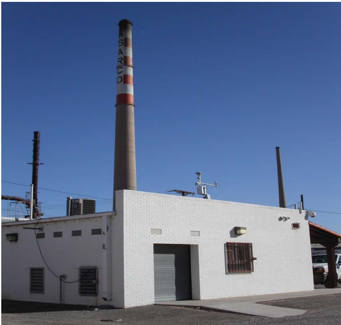
E-BAM #10, International Border and Water Commission Note: The ASARCO stack is no longer active; not emitting particulates
