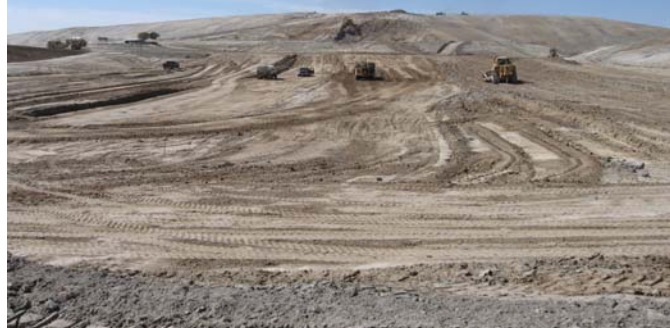
Preparing the area for a landfill liner system at the San Juan County Regional Landfill
