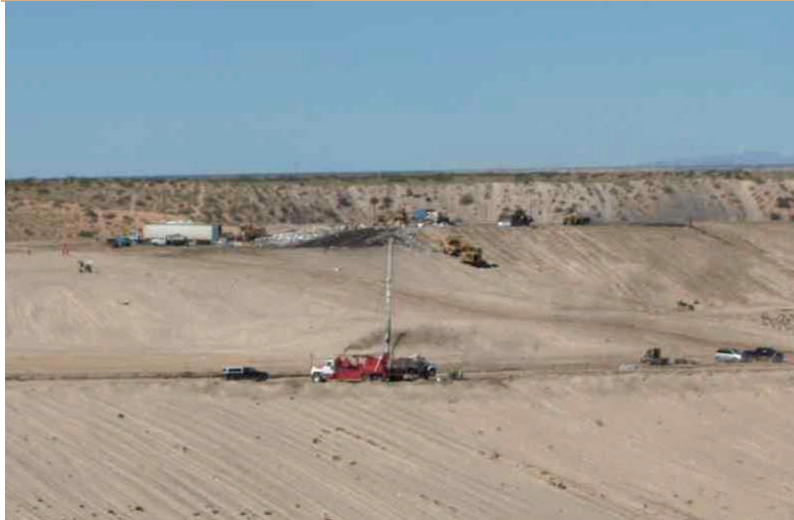
Camino Real Landfill— Installation of a methane gas monitoring well
