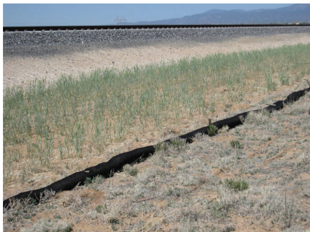
Black filter sock installed along the Rail Runner railway
