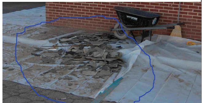
Public health hazard due to the improper demolition and handling of asbestos containing shingles
