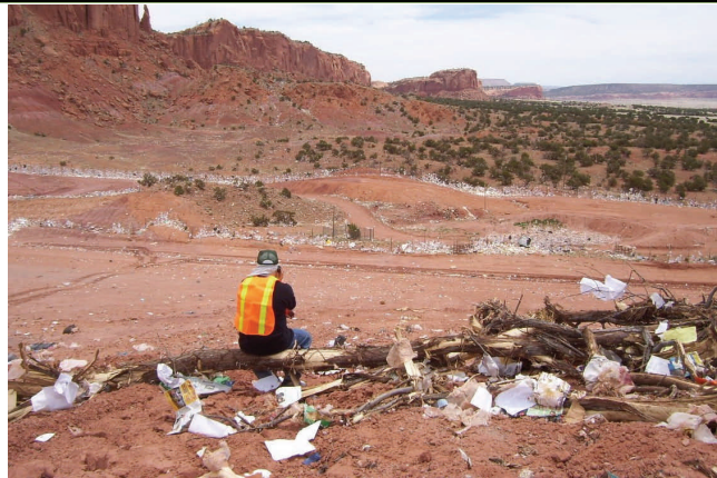
SWB Enforcement Section Manager surveys the blown litter resulting from failure to apply daily and intermediate cover at the landfill
