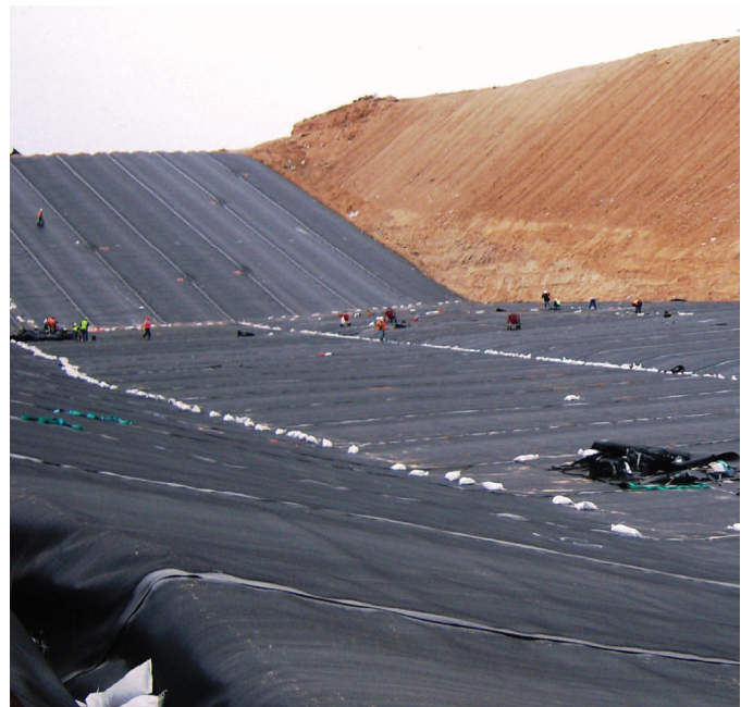
Installation of the protective liner and leachate collection system at the Rio Rancho Landfill
