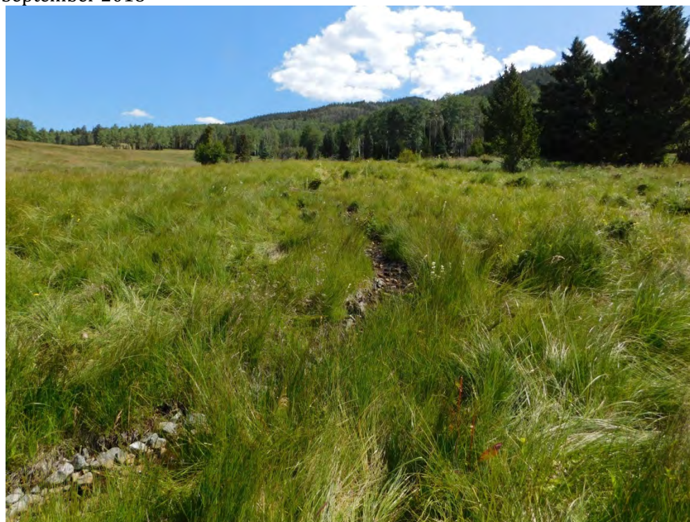
August 2019. Restoration treatment addressed an incised secondary channel through valley wetlands. High banks were collapsed and the new channel profile was armored with angular cobble.
