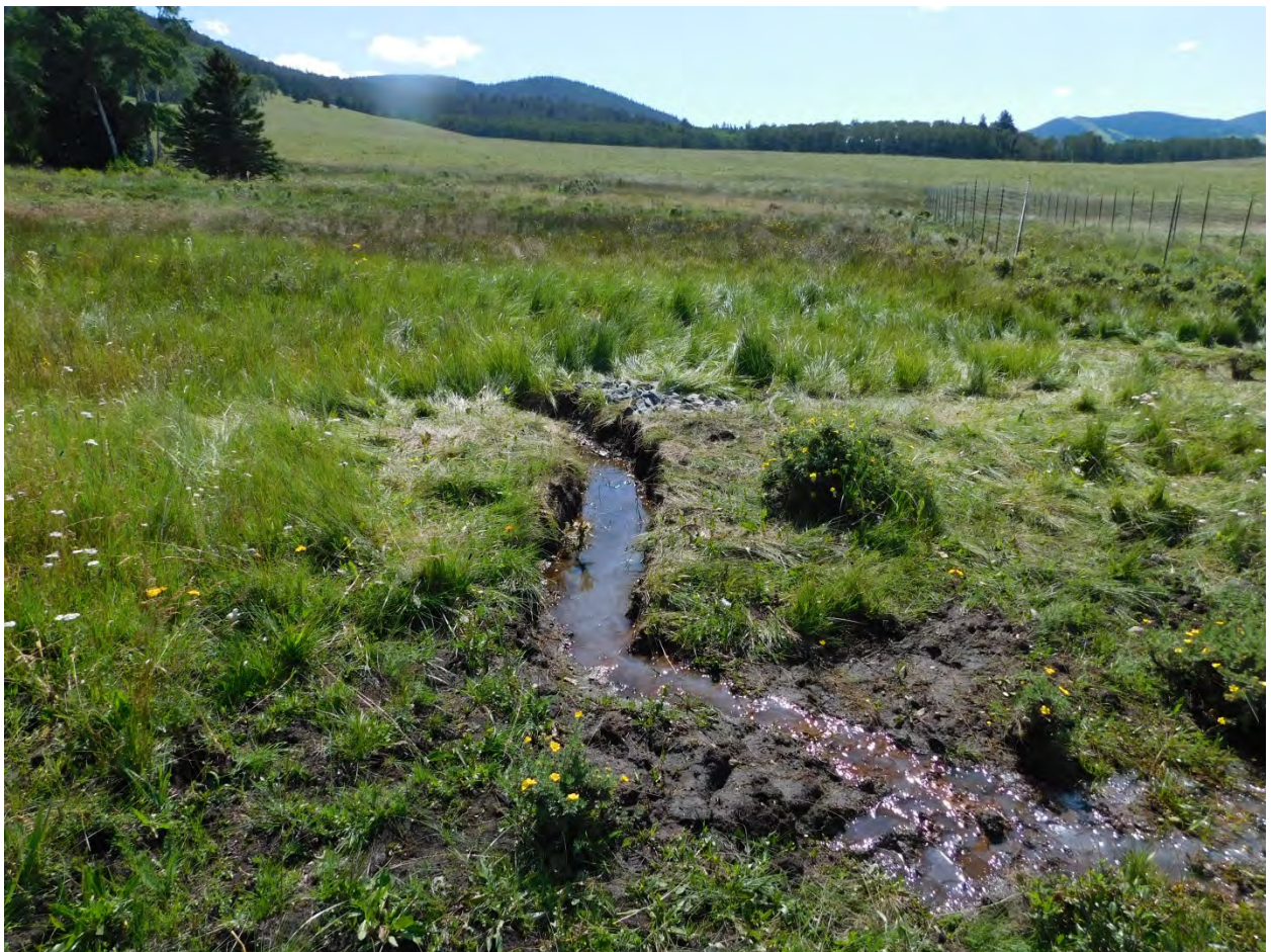
August 2019. Sod swale with rock-armoured stable return
