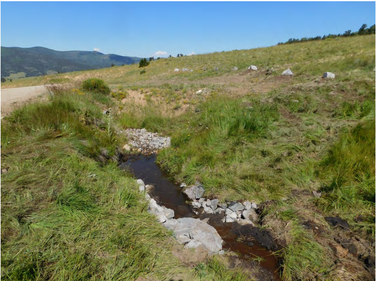
August 2019, Zuni Bowl and rock rundown to stabilize head-cutting and gully formation from Forest Service Road 1950 culvert (2019 NMDGF Funding)
