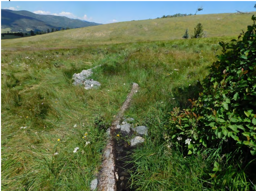
August 2019. Log and rock berm designed to move water toward the center of the valley
