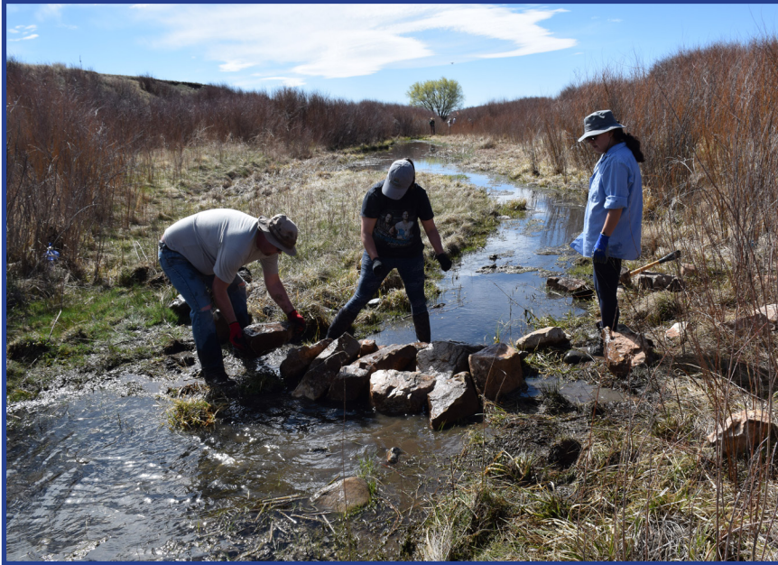
AWF volunteers and HPWA staff building a one-rock dam to raise the grade of Wolf Creek and enhance the adjacent wetlands.
