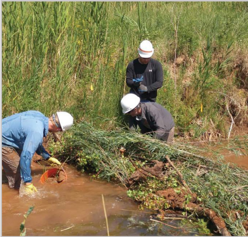
Beaver Dam Analog example provided in a Specification Sheet in New Mexico's FOTG.
