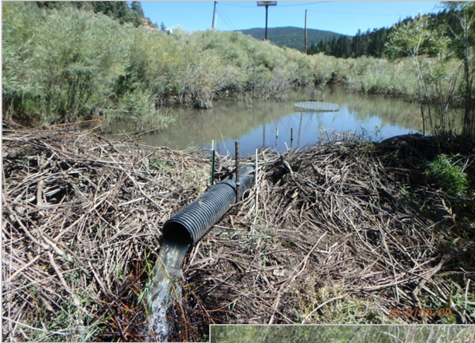
Photo on left. This beaver pond leveler lowered the water level in the pond by about 14 inches, reducing the threat to the county road immediately downstream.
