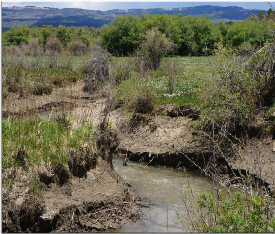
FIGURE 12 RIO NUTRIAS UNSTABLE STREAMBANKS
