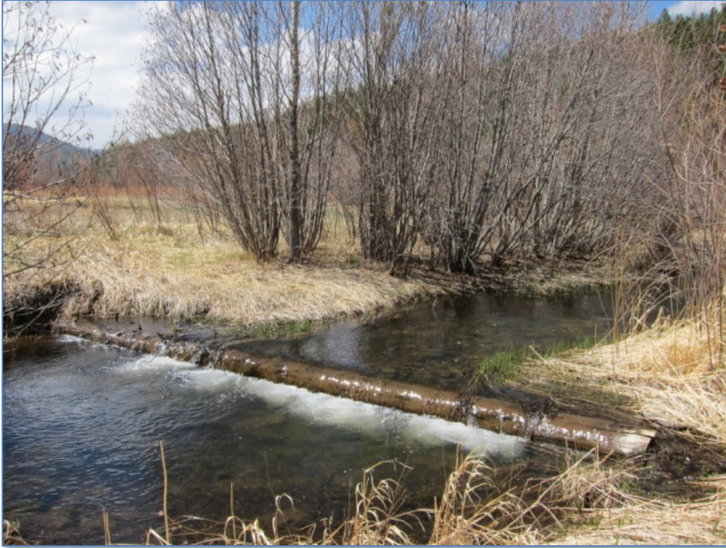
Figure 2 - Channel widening caused by man-made log dam.
