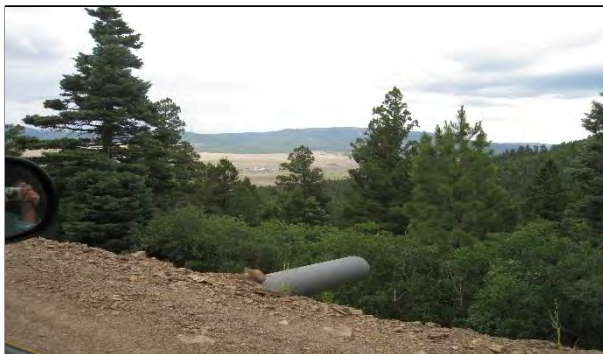
--Poorly placed culverts can accelerate erosion
