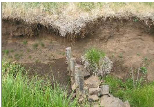
--Post vanes to mitigate bank cutting along Cieneguilla Creek
