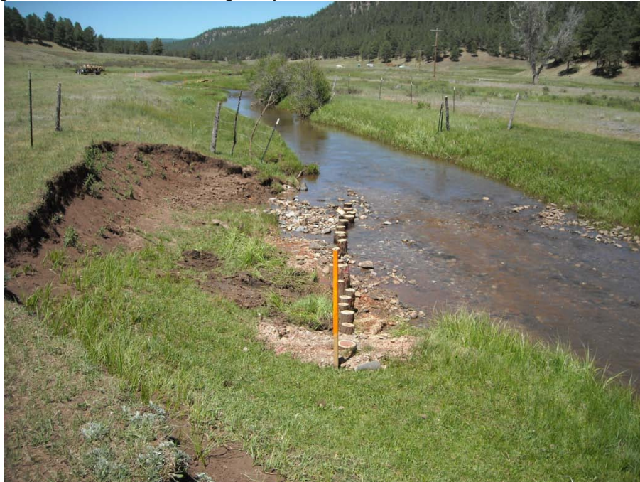
Photo 4. Post vane structure and hemi-fence to protect riparian wetland.
