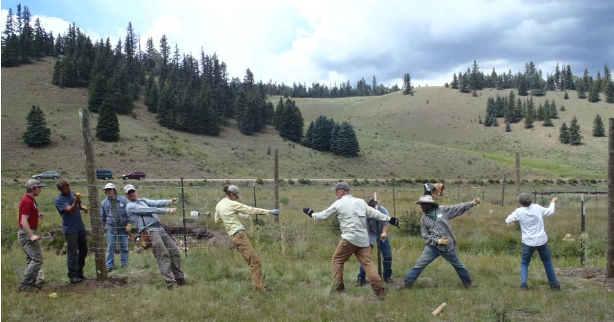
Figure 25. Volunteers repairing elk enclosures to protect willows along Comanche Creek
