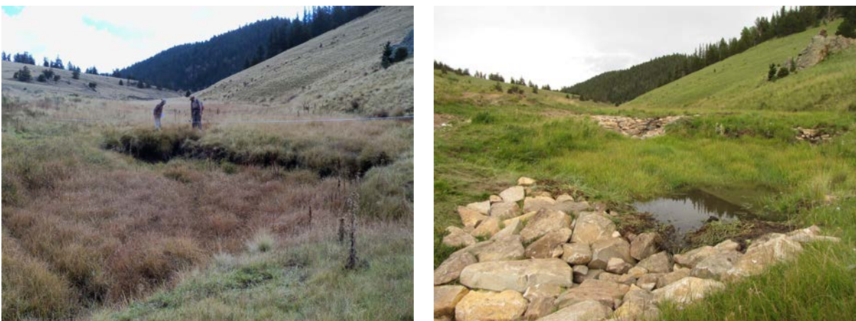
Figure 21a. Cross section measurement of headcut in Grassy Creek; Figure 21b. Zuni bowl remediation of large headcut in 2013.
