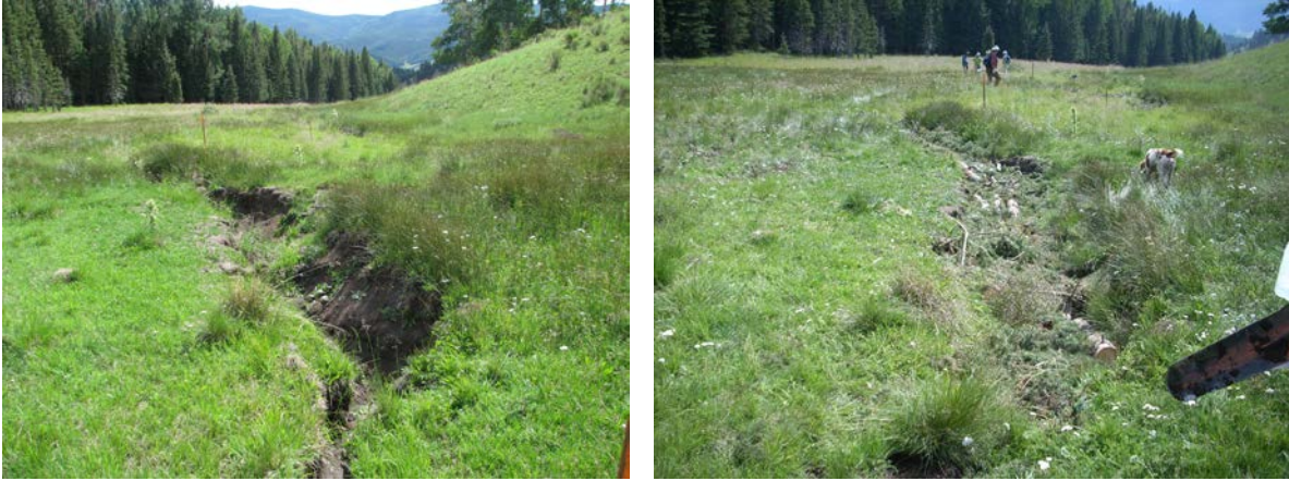
Figure 22a. Smaller headcuts are remediated using logs and sod; Figure 22b shows the headcuts filled with native materials obtained from onsite.
