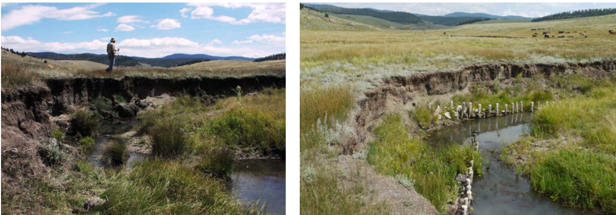
Figure 18a. Erosion and channel incision in the mainstem of Comanche Creek dries the adjacent floodplain and associated riparian wetlands; Figure 18b shows the same area with post vanes installed to stabilize the stream banks.
