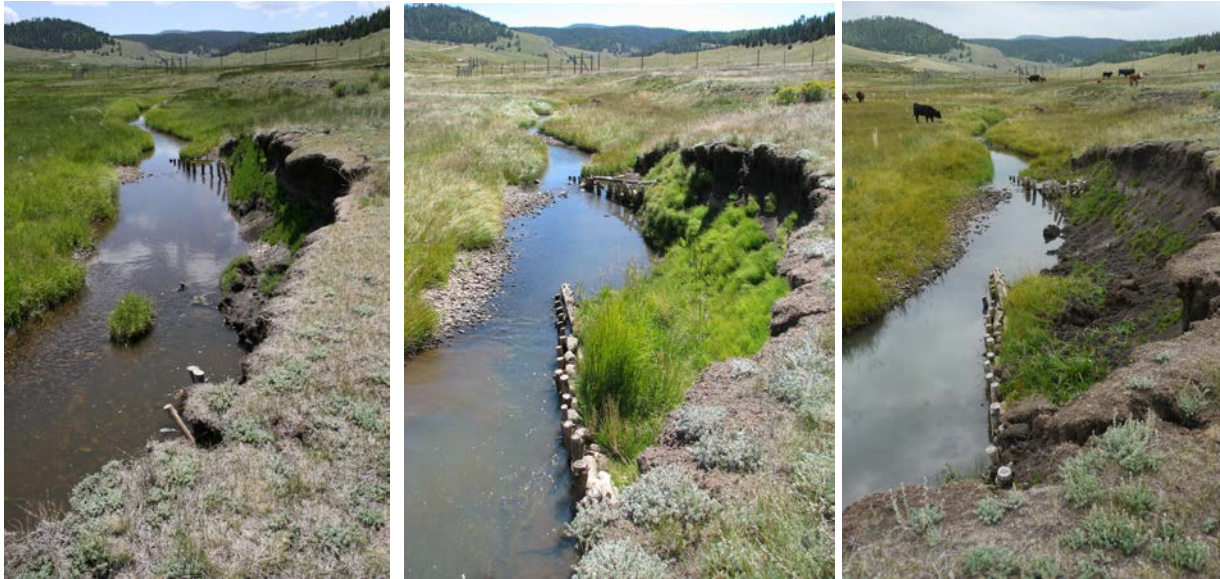
Figure 24. Bank stabilization using post vanes in the Comanche Creek mainstem
