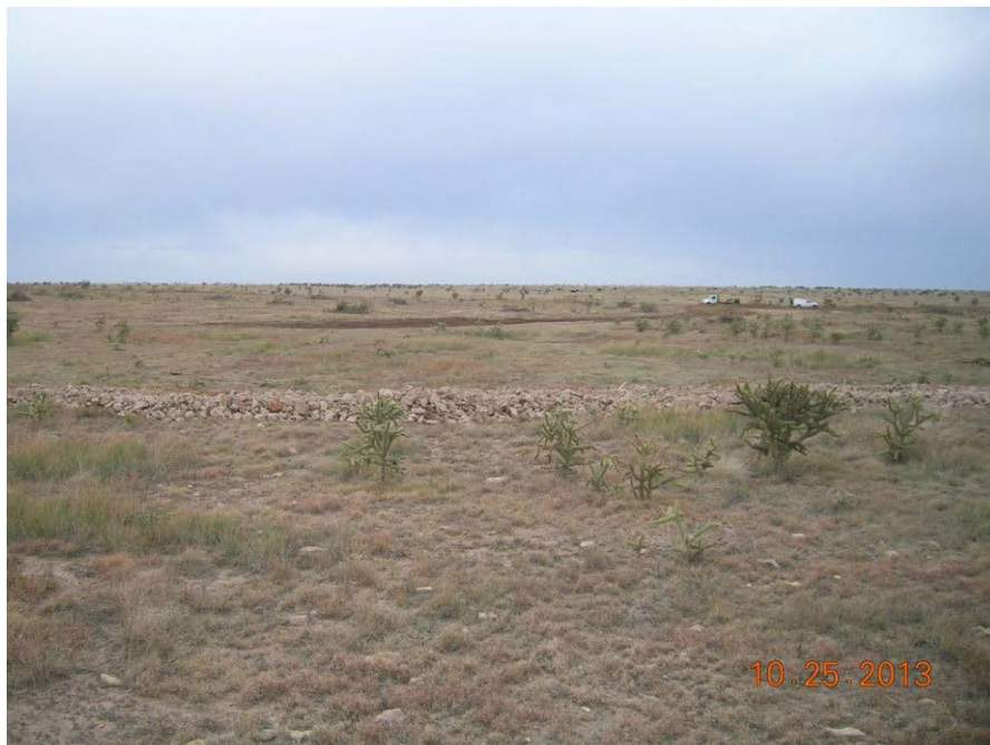
Wood Playa erosion control project - cobble berm in foreground with southern watercourse in background.
