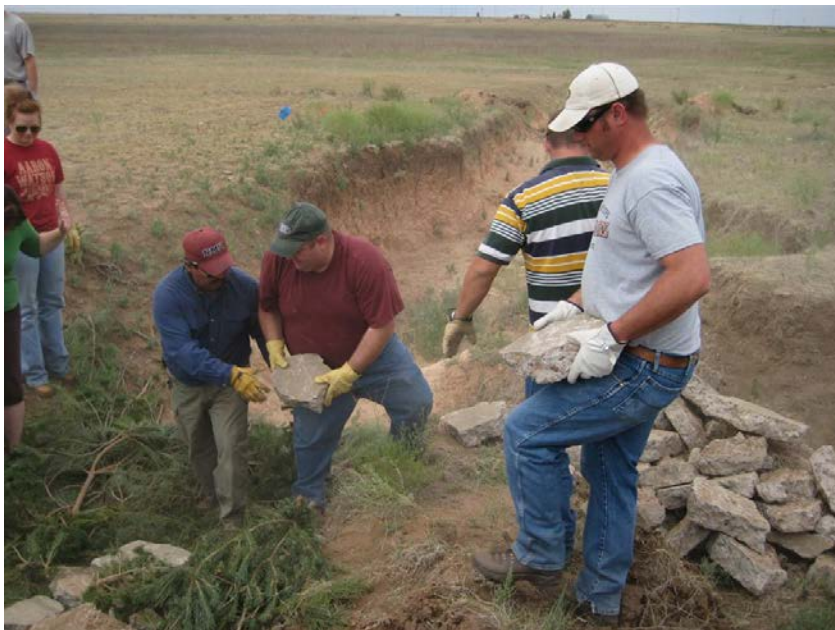
Construction of brush and rock weir structures at an arroyo on Gary Starbuck Playa in June 2009. The volunteers shown are area NRCS staff and TNC staff. The volunteers were organized as part of an NRCS staff training workshop.
