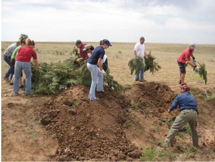
Construction of brush and rock weir structures at an arroyo feeding Jim Starbuck Playa in June 2009. The volunteers shown are area NRCS staff and TNC staff. The volunteers were organized as part of an NRCS staff training workshop.
