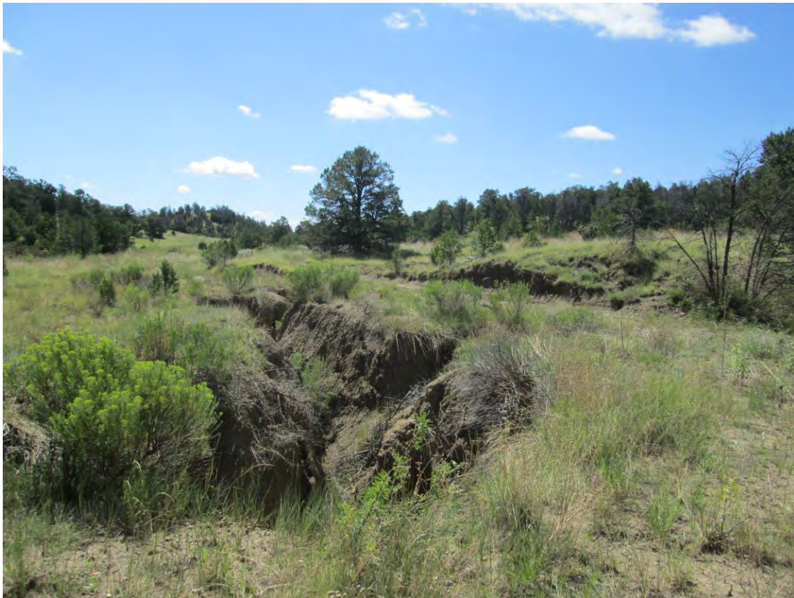
Example of erosional gully resulting from poor road drainage
