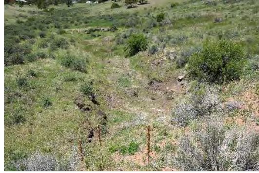
--Presence of shrubby cinquefoil is an indicator of slope wetlands drying below road and culvert
