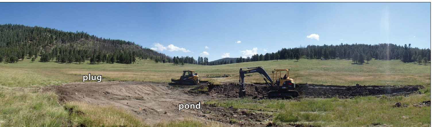
Figure 28. Constructing and compacting the plug. (©S. Vrooman)
