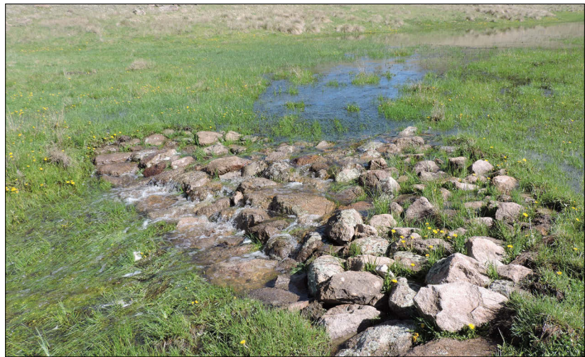
Figure 55. Site 53, May 11, 2017. Rock rundown constructed by volunteers as a stable return site for plug and pond at Site 52. (©W.D. Zeedyk)
