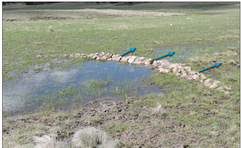
Figure 47. Complex Site 28, May 11, 2017. Media luna spreading water downvalley from plug and pond. (©W. D. Zeedyk)
