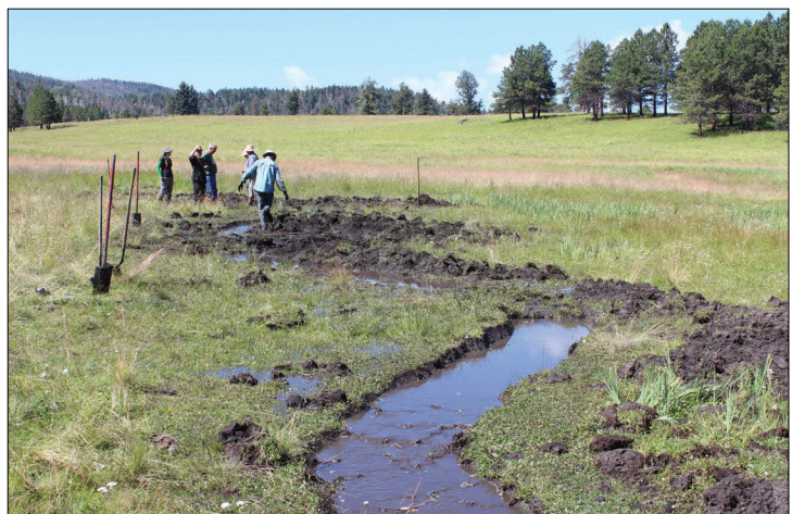
Figure 45. Site 20, July 2015. Worm ditch hand-dug by volunteers. Here water spills as sheetflow to the left. (©K. Menetrey, NMED)
