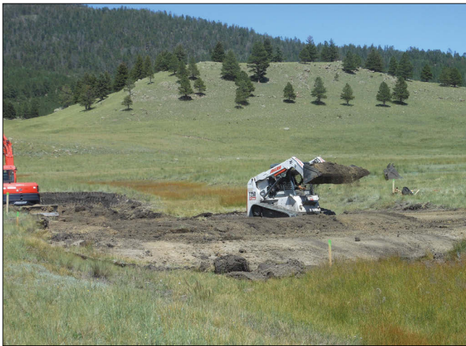
Figure 36. Tres Arroyos, August 2012. Left, skid loader adds fill dirt excavated from the pond to the surface of the plug. Right, sod tiles stockpiled prior to constructing the plug are placed on the completed plug. (©S. Vrooman)
