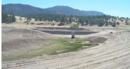
Gradient and sediment control structures.
