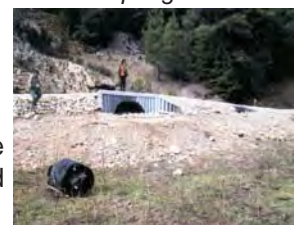
Constructed culverts to direct spring water.
