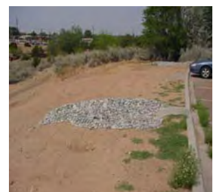
Cobble basins at outlets of the Oliver Lafarge Library parking lot are highly visible to library patrons and motorists on nearby Siringo Street.
