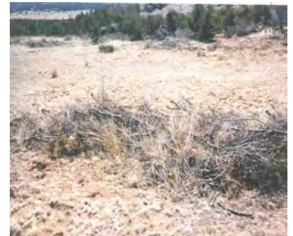
Vegetative growth after bundle placement in Abo Arroyo.
