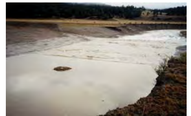
Sediment collecting in sediment control structure.
