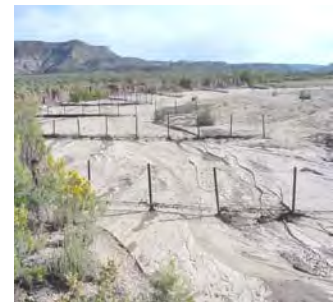
Completion of the Riparian Sediment Retentions Fences in Carrizo Wash.
