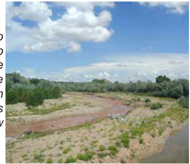
Galisteo Creek repositioned to a mid-channel area to keep shear pressures off the receding bank, and the detention berm with built-in rock vane structures is beginning to establish new
