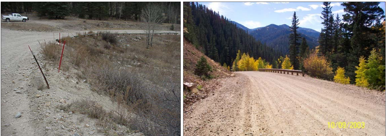
Malette Road before reconstruction (left) and after reconstruction (right).
