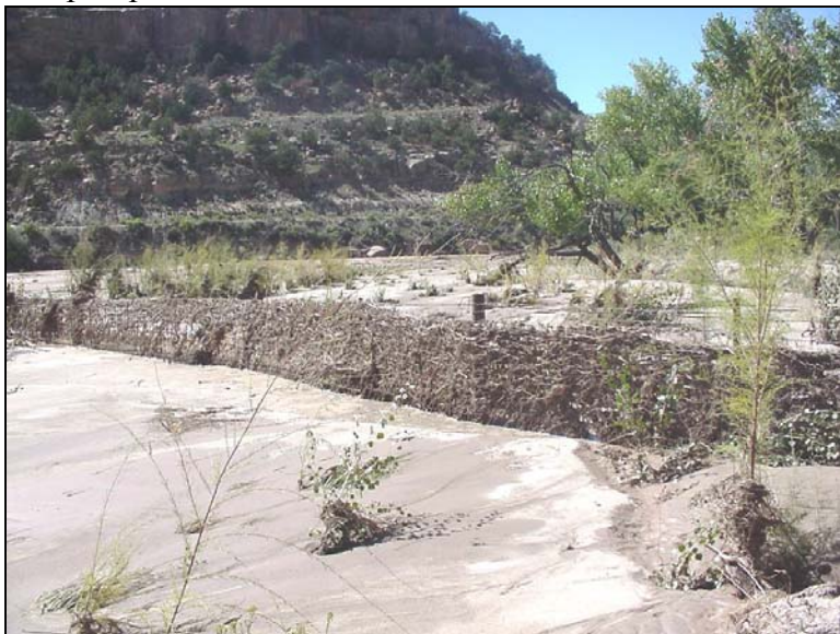
Carrizo Canyon sediment fence.
