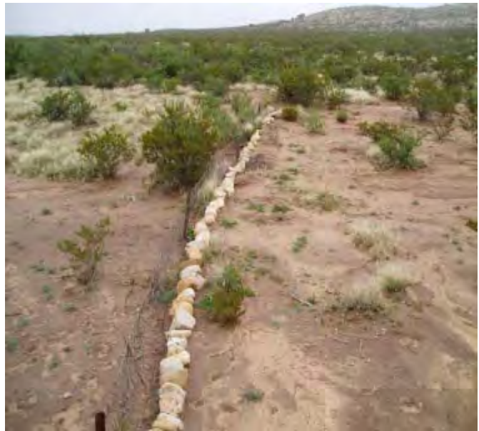
Sediment retention fence at Big Hackberry, designed to slow flow and trap sediment. Completed June 2004
