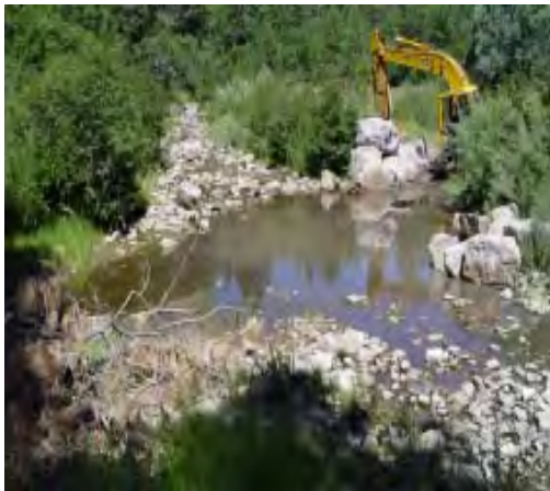
Before picture of the lower ford. Excavator was just staging the rock on the bank.
