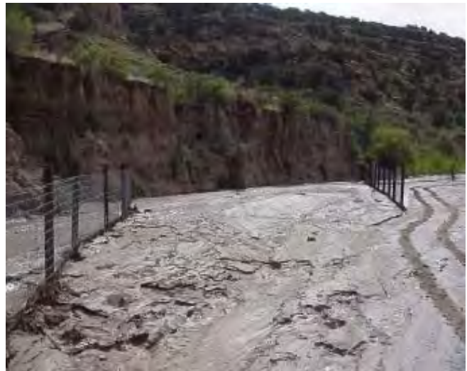
Recently installed sediment fence demonstrating protection of eroding stream banks and riparian vegetation.
