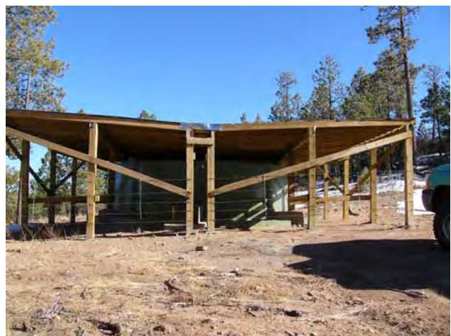
Trick Tank constructed to draw livestock and wildlife from riparian areas of Rio Gallina.
