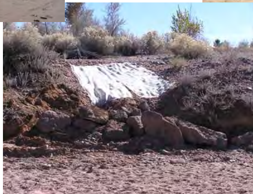
Erosion control seed mat and boulders placed to minimize erosion.
