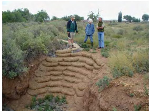
A sand bag erosion control technique: Large jute bags, filled with partly decomposed wood chips and on-site dirt, native seed mixes (jute-bag technique developed & tested at EWI ranch in 2004 & 2005—applied at 2 demonstration sites. Promises to be effective, but needs to be tested and monitored for several years to prove long-term viability.
