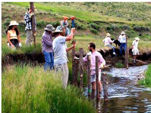
NM Trout volunteers installing vane structure in Comanche Cr. during a work weekend.
