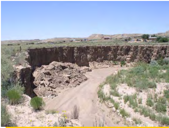
Rio Puerco near Cabezon: Mass failure of a 35-foot high arroyo wall into the active channel.
