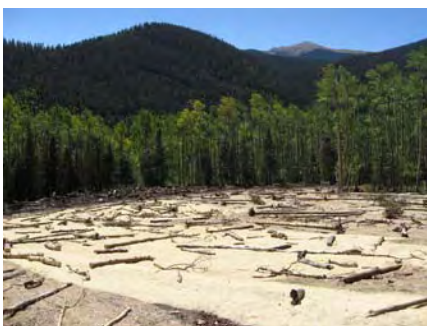
Placer Creek consolidation cell – final grade with erosion control measures in place.
