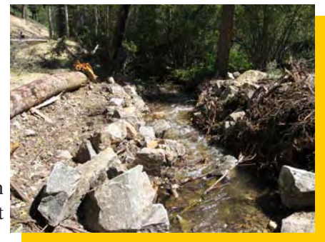
Streambank re-constuction utilizing rock and root wads at Midway Tunnel Prospect.
