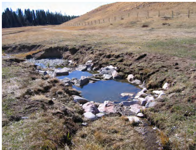
Zuni bowls on Placer Creek to mitigate erosion.
