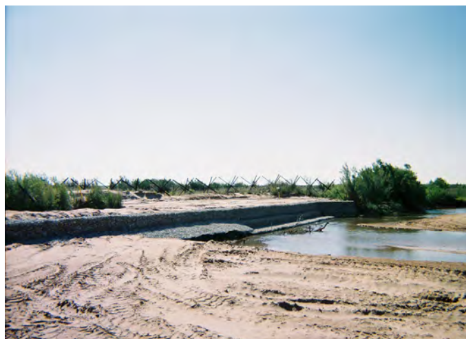
Bank stabilization on the Pecos River.
