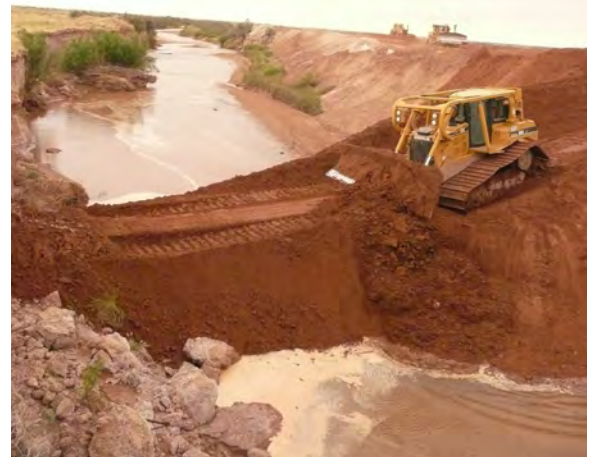
Plugging the Pecos River prior to re-connecting Oxbow 4.
