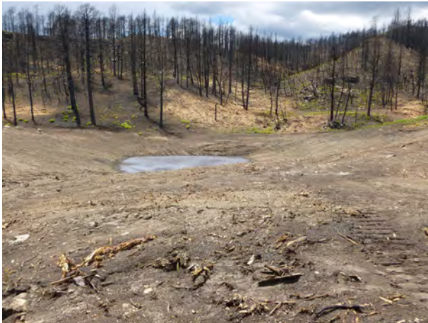
A sediment retention basin constructed above Lake Maloya.
