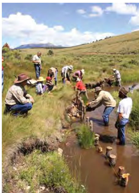
Volunteer crew constructs post vane in Comanche Creek to mitigate stream bank erosion.
