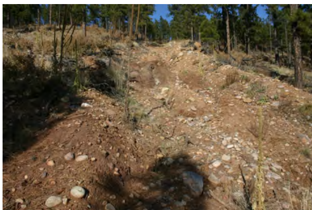
Road prior to reclamation to reduce sediment runoff.
