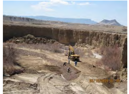
Project under construction.
