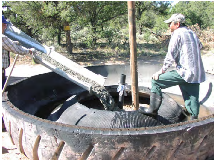
Construction of a "large tire" drinking trough.
