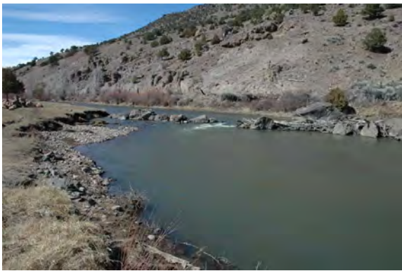
Failed irrigation diversion structure and associated bank erosion.
