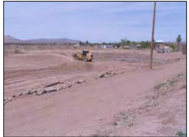
Heavy equipment excavating and shaping the future La Mancha Wetland. Photo courtesy of Southwest Environmental Center.
