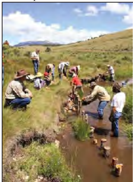
Volunteer crew constructs post vane in Comanche Creek to mitigate stream bank erosion.
