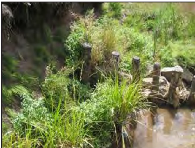
A post vane constructed on Cieneguilla Creek to divert high velocity flow away from a cutbank. Photo courtesy Cimarron Watershed Alliance.
