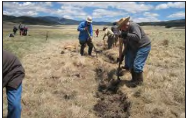
Project volunteers from Los Amigos de Valles Caldera dig and haul sod to form a channel plug. Photo by Karen Menetrey, NMED.
