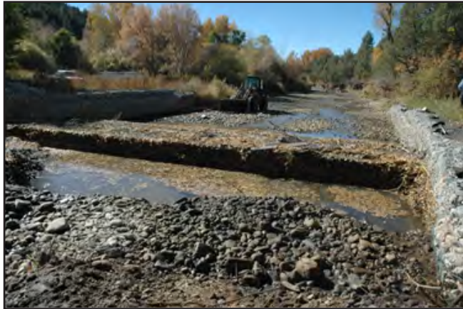
Project area before restoration, looking downstream at the old gabion dam in the west channel. Photo courtesy of Upper Pecos Watershed Association.
