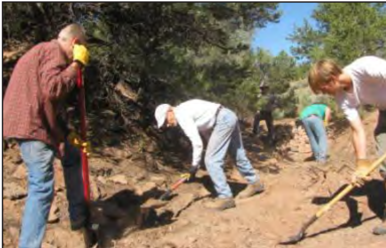
Community work event at Galisteo Creek in October 2010. Volunteers are building rock structures for erosion control. Photo courtesy of EarthWorks Institute.
