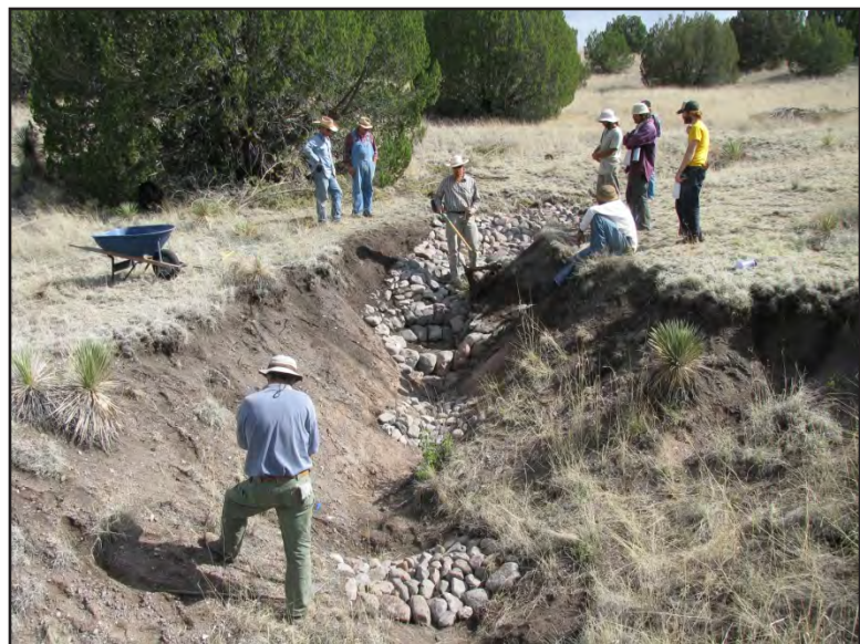
Cold Springs Gully Rehab Workshop May 2009
