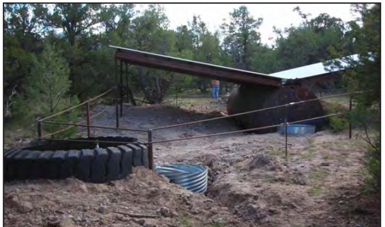
Completed trick tank
