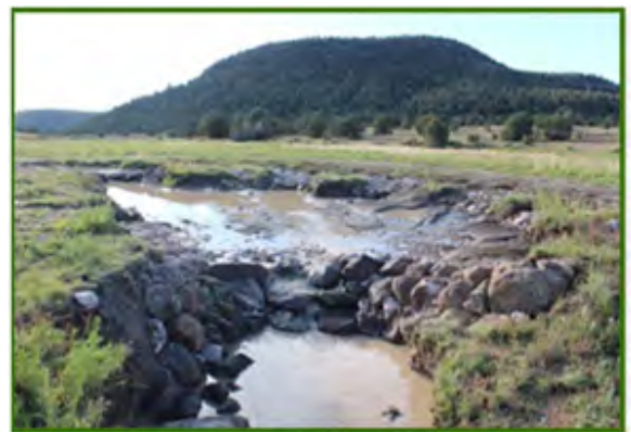
Before (top), during (middle), and after (bottom) construction of a Zuni Bowl to arrest headcut migration that was draining valley wetlands.
