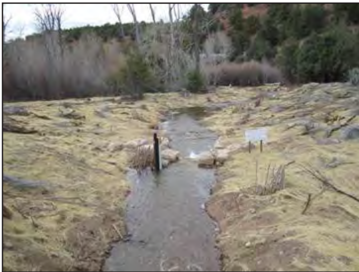
The new Santa Fe River channel, immediately following construction and planting. Photo by Santa Fe Watershed Association.
