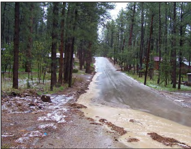
Sediment laden stormwater.
