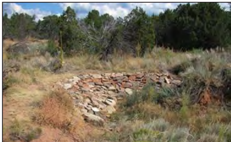
A media luna rock structure constructed at Galisteo Creek to disperse flow. Photo courtesy of EarthWorks Institute.
