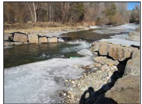
Cross vane on the Pecos River reduces erosion and creates fish habitat.
