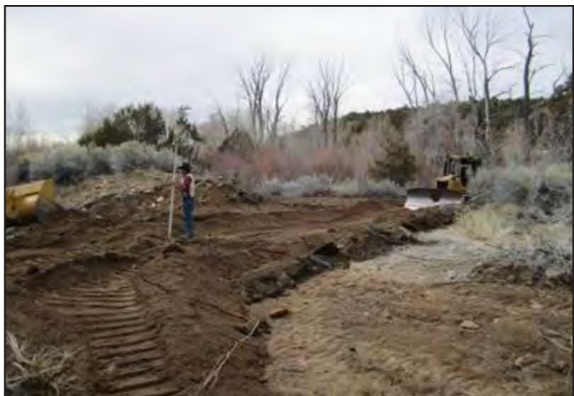
Contractor Steve Carson, Rangeland Hands, during construction of Santa Fe River Channel. Photo by Santa Fe Watershed Association.
