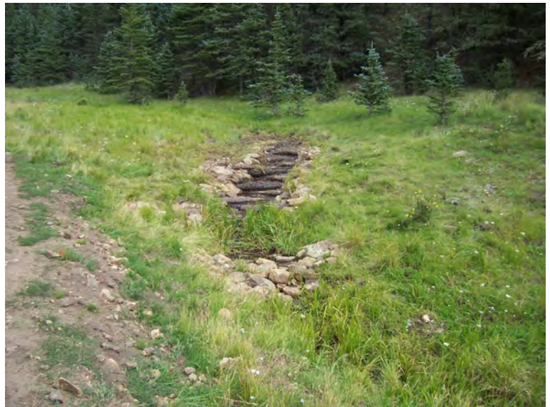
Stream restoration structure addressing a headcut in Grassy Creek requiring a NWP 27 for Aquatic Habitat Restoration, Establishment, and Enhancement Activities.
