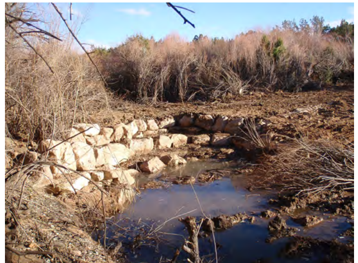
Headcut restoration structure constructed at San Marcos by Rangeland Hands, Inc.
