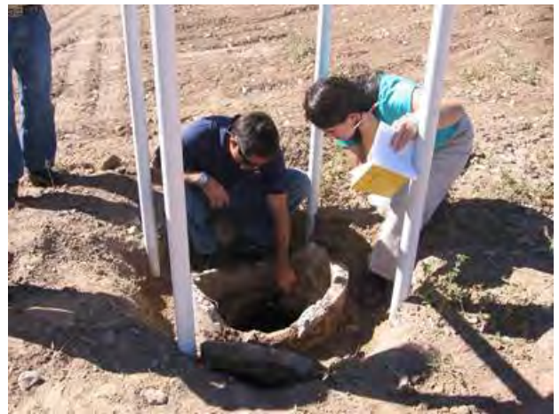
GWQB staff inspecting a septic tank at the Santa Fe Equestrian Center.
