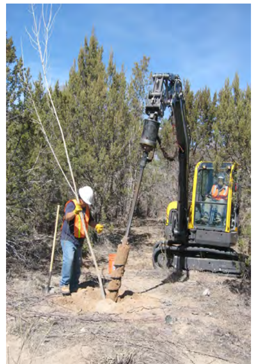
Holes were augered eight feet to groundwater to plant cottonwood poles.
