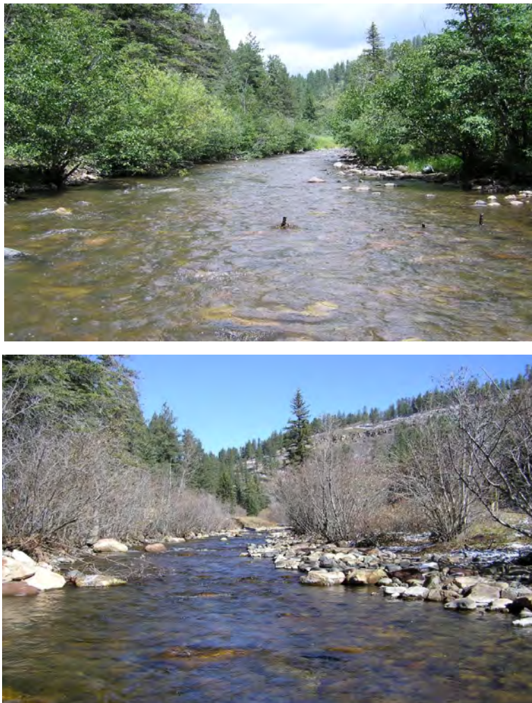
Figure 2. Pre-construction (upper) taken in August 2012 and post-construction (lower) taken in October 2013 at photo point MP2 looking upstream. Even though flow was lower in October 2013, deeper pool habitat is present in the lower left of the photo.
