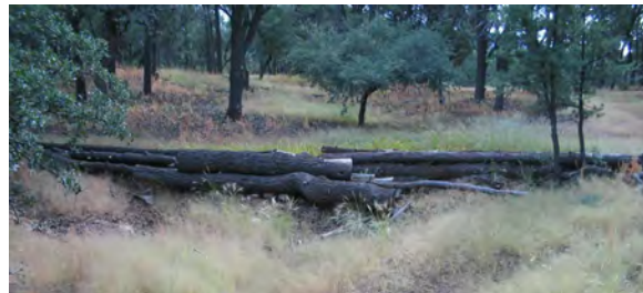
Log Erosion Control Structure.
