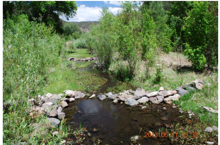
Two of the hand constructed rock weirs in Black Canyon that focus streamflow to encourage scour pool development, enhance fine sediment deposition and riparian vegetation recruitment.
