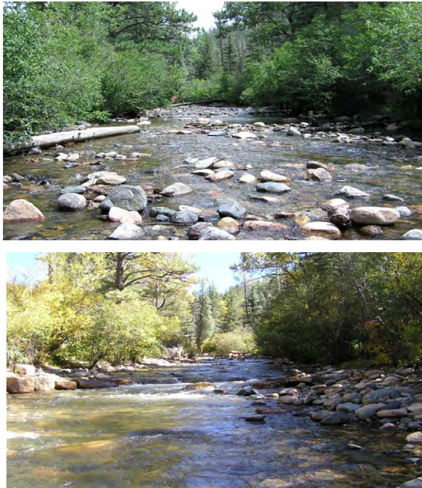
Figure 1. Pre-construction (upper) taken in August 2012 and post-construction (lower) taken in October 2013 at photo point MMI looking upstream.
