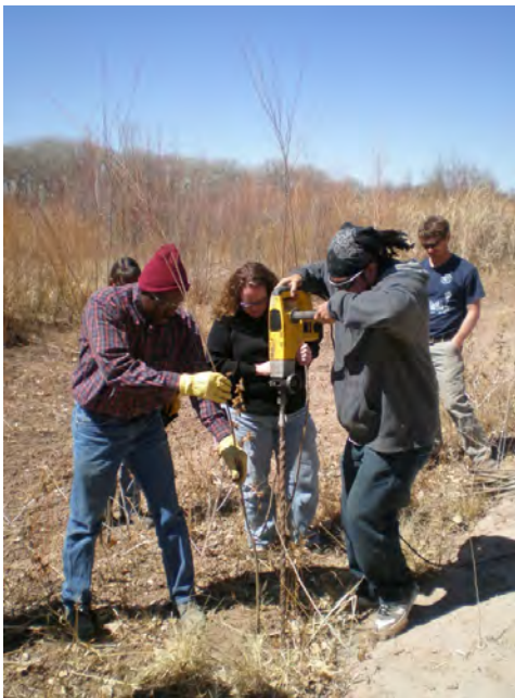
Participants at a planting workshop using a rotary air hammer to drill holes for planting willows on State Trust Land bosque.
