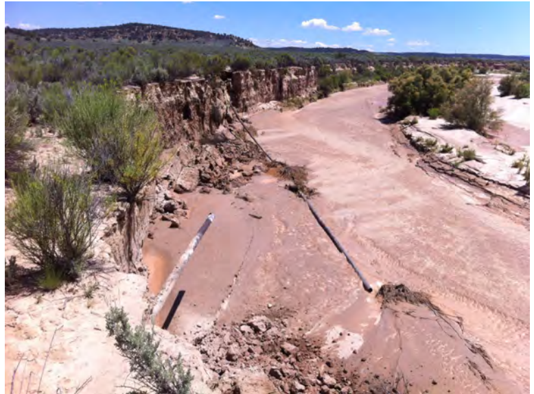
A broken natural gas pipeline in Largo Wash following a thunderstorm in August, 2014. Subsequent repair and bank stabilization was authorized under the Section 404 Regional General Permit for Activities in Emergency Situations.
