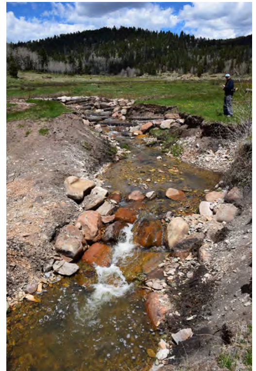
A series of grade control structures were installed to reduce erosion and halt headcut migration into the meadow on Placer Creek.
