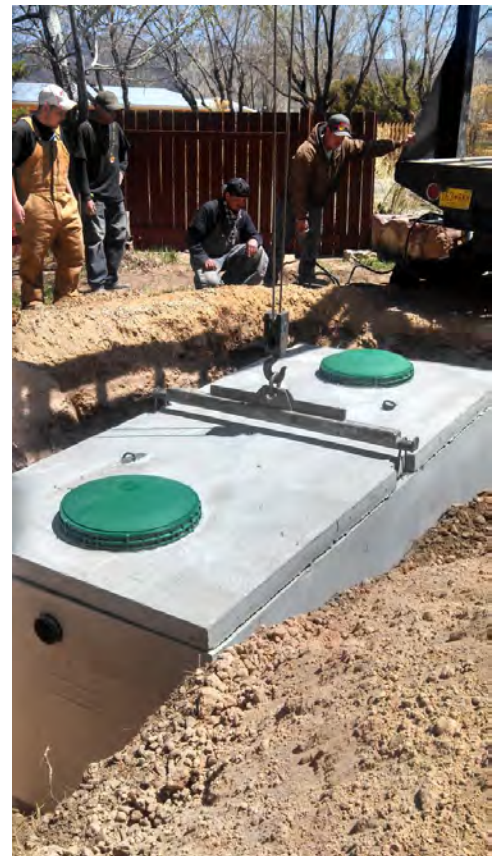
Installation of a new septic tank permitted by the GWQB at Pagosa Hills Mobile Home Park.
