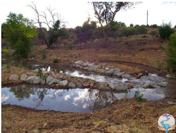
A new cross-vane shown during a moderate flood event. The cross-vane prevents erosion down to a sewer line that had been damaged by prior flooding.
