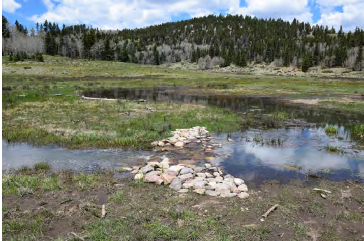
A flow splitter was installed that inundates the meadow during higher flows reducing erosion, storing water and improving habitat.
