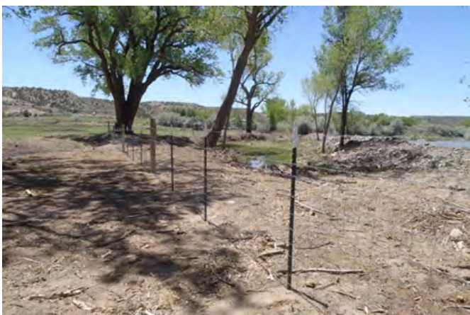
Riparian fence on the Blancett farm along the Animas River on 5/22/13 right after Russian olive removal and fence installation.
