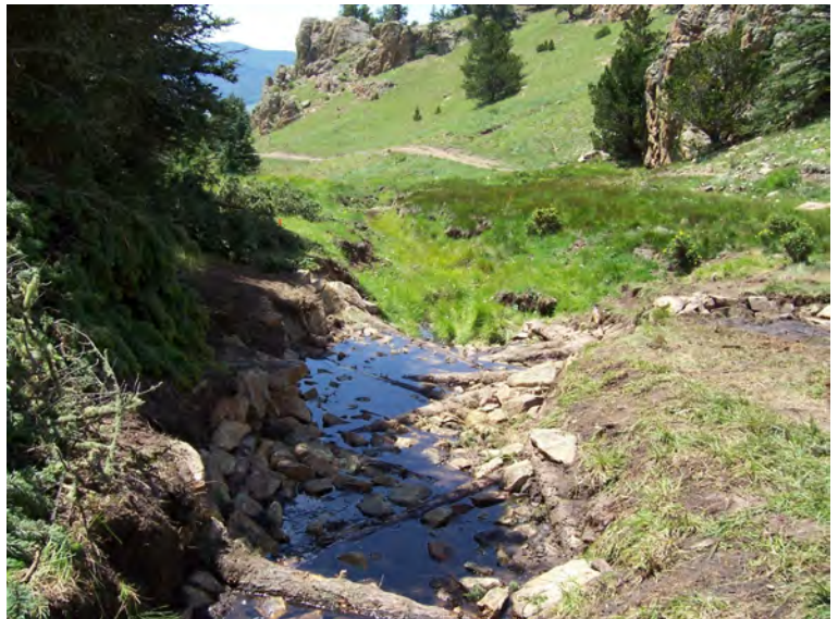
Head cut in lower Grassy Creek, Valle Vidal after treatment with a machine built log and rock rundown structure. This structure will hold the grade and help prevent the de-watering of upstream slope wetlands.
