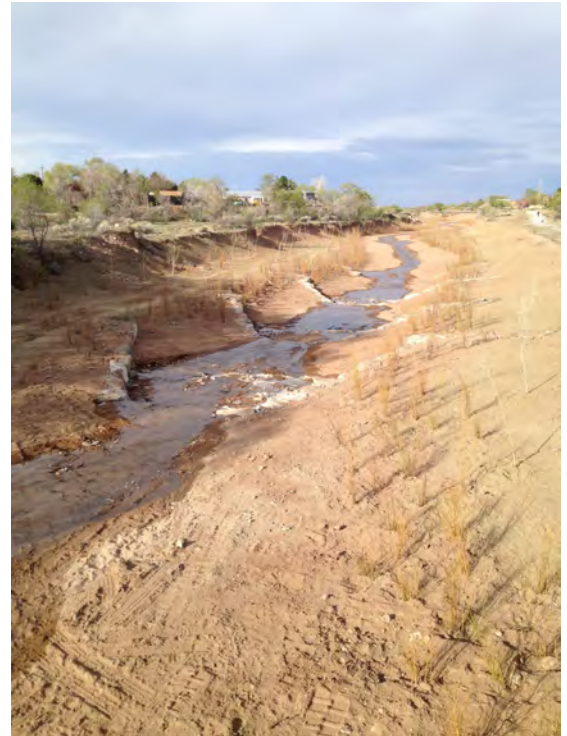
Crossvanes and willows installed along the Santa Fe River under NWP 27 for Aquatic Habitat Restoration, Establishment, and Enhancement Activities.
