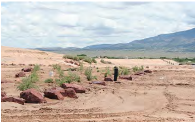
Newly installed rocks and willows designed to filter sediment, and collect la ge debris to reduce pollutant loading to the Rio Grande.
