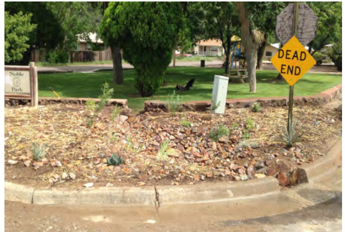
Before (right) and after (left) photos of a completed stormwater harvesting basin at Noble Park in Silver City. Stormwater flows from the left through the curb cut into an infiltration basin. Excess water flows through the wall cut in the background to irrigate park vegetation.
