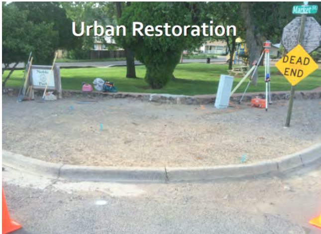
Before (right) and after (left) photos of a completed stormwater harvesting basin at Noble Park in Silver City. Stormwater flows from the left through the curb cut into an infiltration basin. Excess water flows through the wall cut in the background to irrigate park vegetation.
