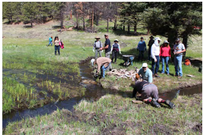
Volunteers install one-rock dams and cobble run-downs to stabilize a recently built water spreading structure on the valley bottom of upper Jaramillo Creek (May, 2015).
