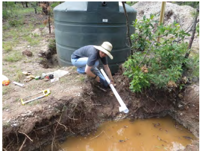
A water catchment system was built for a Gallinas landowner away from the stream to reduce soil compaction and erosion in the riparian area.
