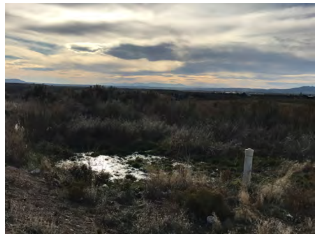
Inspection of a permitted septic tank/leachfield system reveals corrective actions are required.
