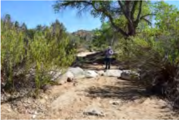
Constructed rock cross vane prevents head cuts from migrating upstream.
