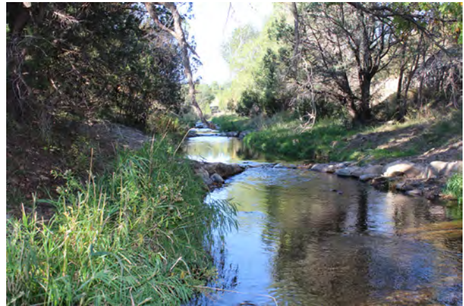
A series of cross vanes in the Rio Ruidoso permitted under NWP 27 for Aquatic Habitat Restoration, Establishment and Enhancement Activities.
