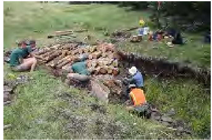
Grassy Creek (left) and Springwagon Creek (right). Volunteers building log step fall structures to arrest erosion in head-cuts, preventing the slope wetlands upstream from drying.
