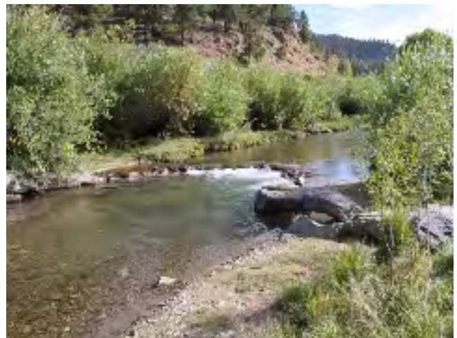
Cross vane constructed at the Red River Westside Fishing Park controls the grade, aerates river water, and provides fish habitat.
