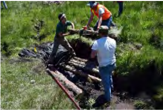
Grassy Creek (left) and Springwagon Creek (right). Volunteers building log step fall structures to arrest erosion in head-cuts, preventing the slope wetlands upstream from drying.
