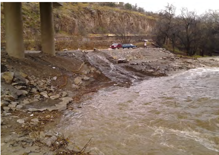
Runoff flowing off a dirt parking lot into San Vicente Creek in Silver City, New Mexico.
