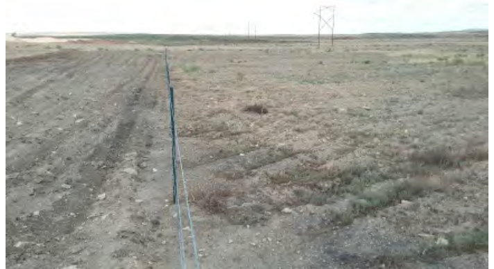
At the Brie I mine, newly completed earthwork is shown to the left of the fence compared to two-year old reclamation work on the right.
