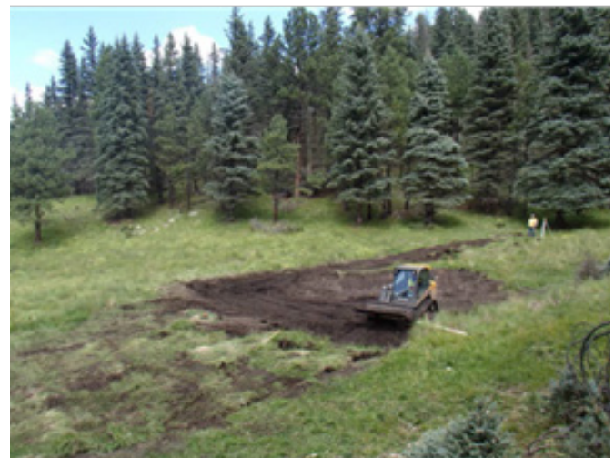
Machine construction of a plug and pond structure along Sulphur Creek.
