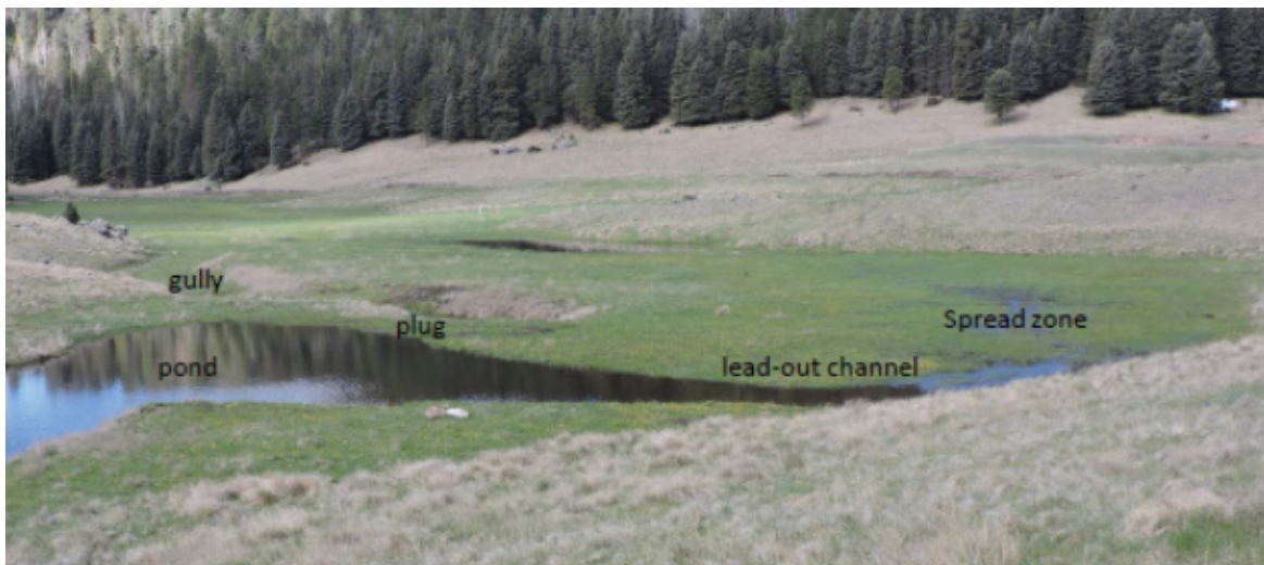
Key features of a typical plug and pond structure (From: Zeedyk and Vrooman 2017)
