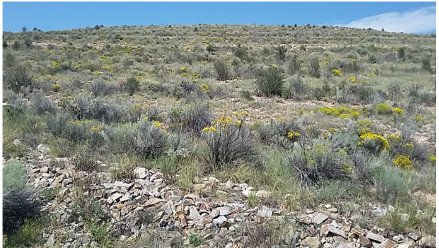
A rock-lined drainage network at the base of a hill, terracing on the hillslope, and successful revegetation efforts promote soil stability at the Cunningham Hill Mine.
